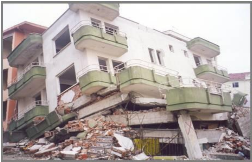
Figure 2.8: Damage due to a soft story at the ground floor during Izmit earthquake in Turkey (1999) [14]
