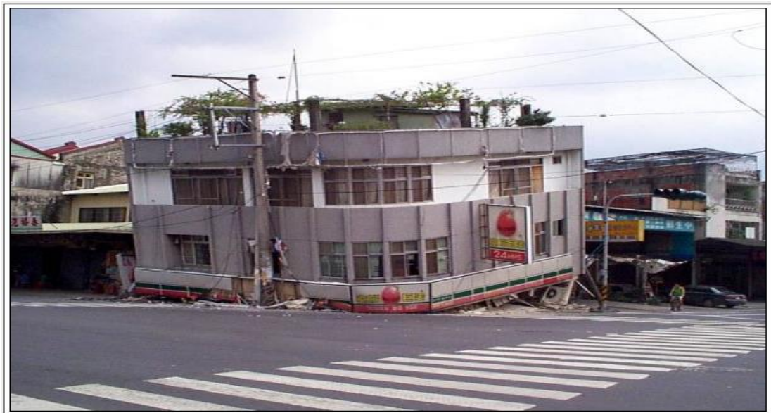
Figure 2.7: Damage due to a soft story at the ground floor during Chi-chi earthquake in Taiwan (September 21, 1999) [13]
