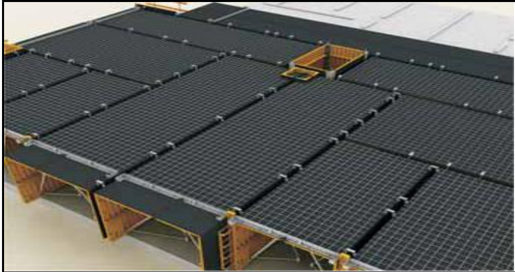
Figure 2.12: Installation the Reinforcement on the Formwork (URL9)
