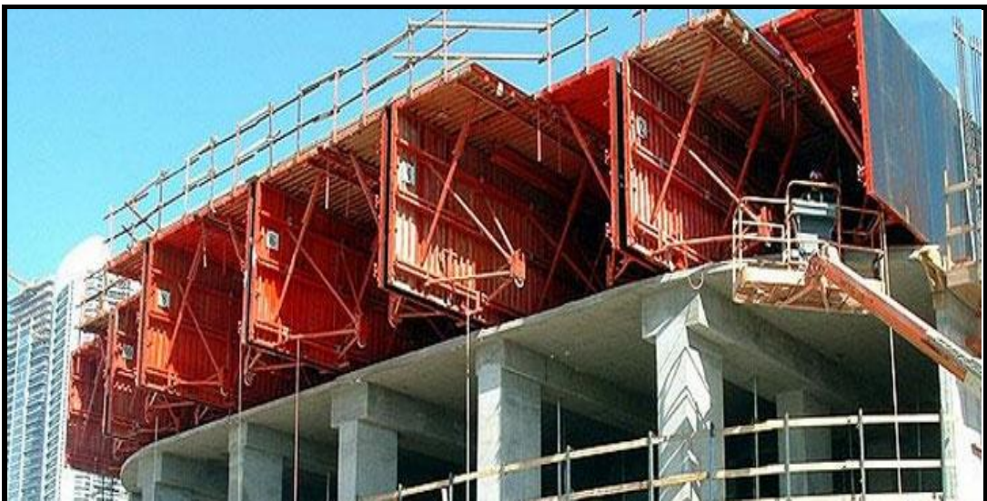
Figure 2.21: HRTF Tunnel Formwork (URL5)
