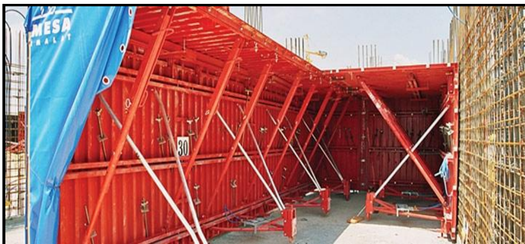
Figure 2.18: ERTF Tunnel Formwork (URL5).
