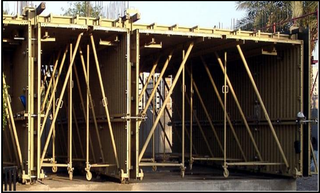
Figure 2.19: TRTF Tunnel Formwork (URL5).
