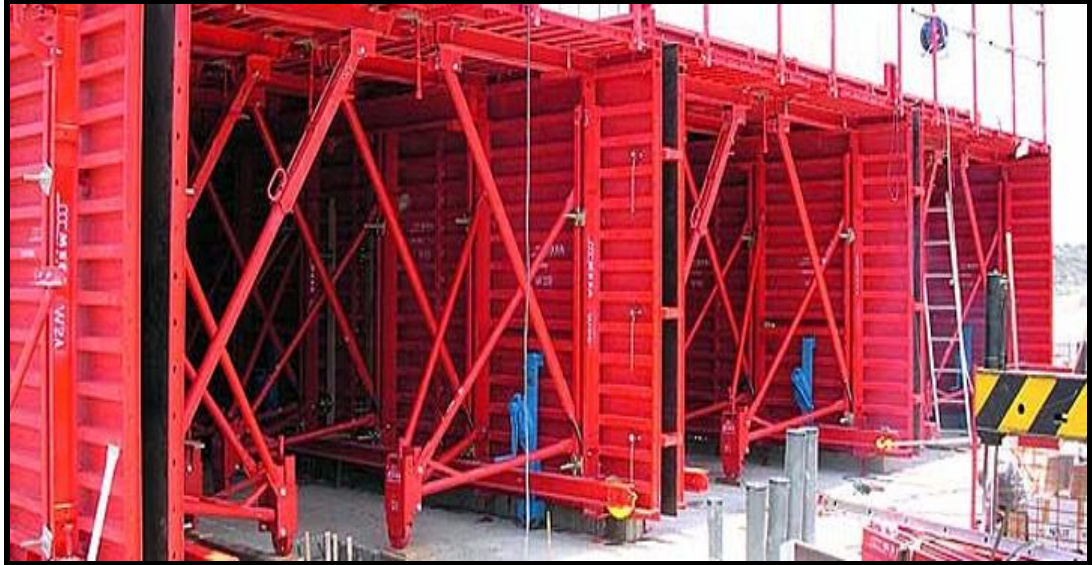
Figure 2.20: NLTF Tunnel Formwork (URL5)
