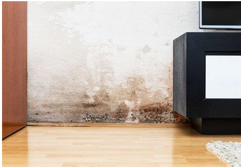
Figure 5: Signs of molds and dampness due to indoor pollutants (Molhave, L. 2008)
