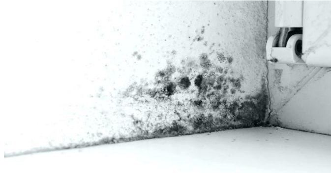
Figure 7: Signs of molds and bacteria which causes to bad odour (Gallego, E., Roca. 2009)
