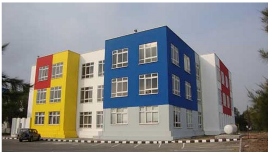
Figure 15: EMU Colored Building (Taken by Author)
