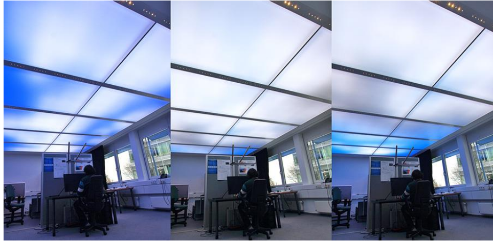
Figure 9: LED ceiling to simulate the sky and satisfy occupant circadian rhythms (Begemann, S. H. A.1997)
