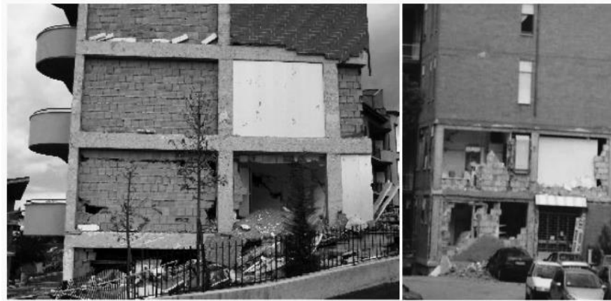
Figure 2.8: Out-of-plane infill wall failure after the Abruzzo, Italy earthquake [1, 23].
