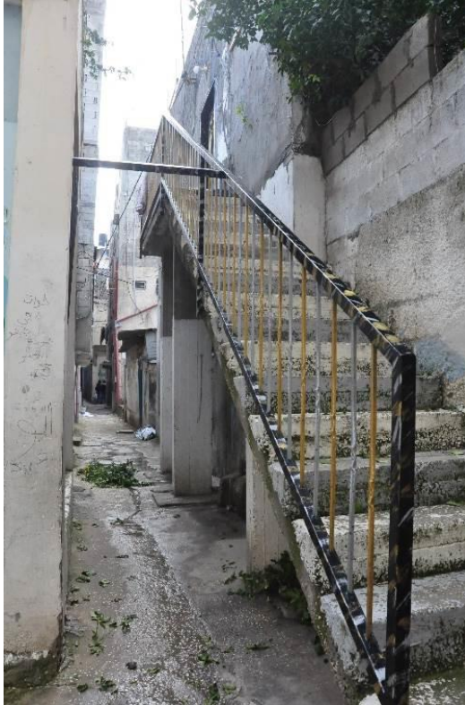
Figure 21: Stairs in the alleys of refugee camp
