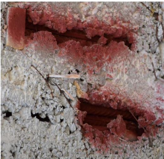
Figure 3.10: Visible Voids around Reinforcements Due to High Congestion. Residential Building, Mağusa, North Cyprus. (Case Study #104 (Page 196)).
