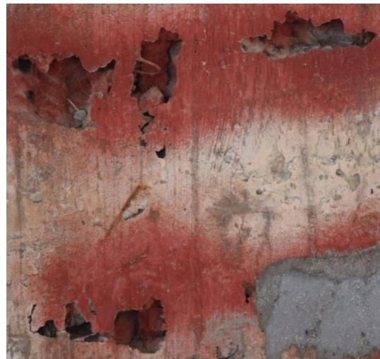
Figure 3.10: Visible Voids around Reinforcements Due to High Congestion. Residential Building, Mağusa, North Cyprus. (Case Study #104 (Page 196)).
