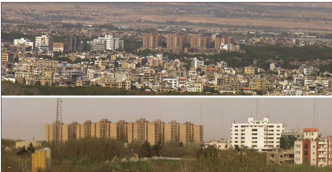
Figure 15. Mortafa Housing - Urban views to the complex. Source: Author
