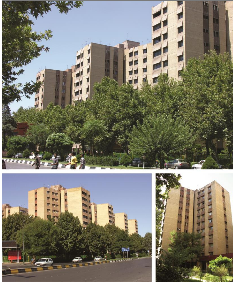
Figure 16. Mortafa Housing Complex - Views to the project. Source: Author
