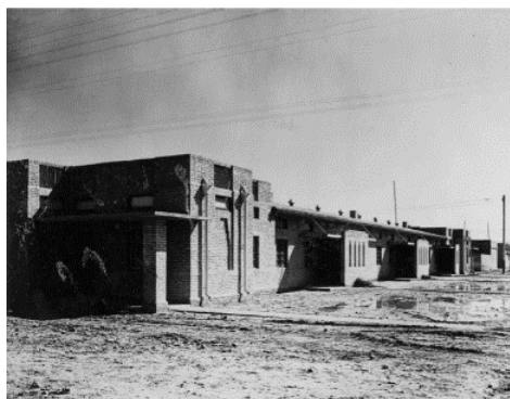
Figure 26. Housing at Bahmanshir, Abadan, 1950 (Photos: Wilson Mason & Partners)
