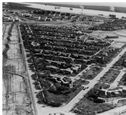
Figure 28. Bawarda, Abadan, 1950 (Photos: Wilson Mason & Partners)
