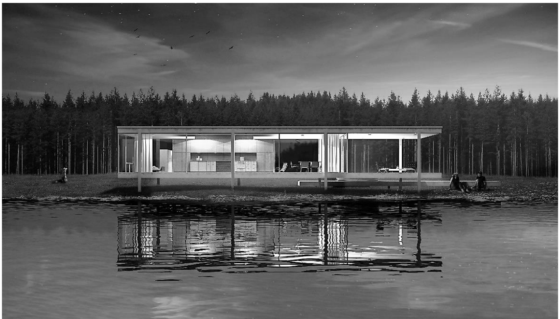
Figure 106. The Farnsworth House Has Been Flooded Considerably Twice Till Now (Clemence, 2006)
