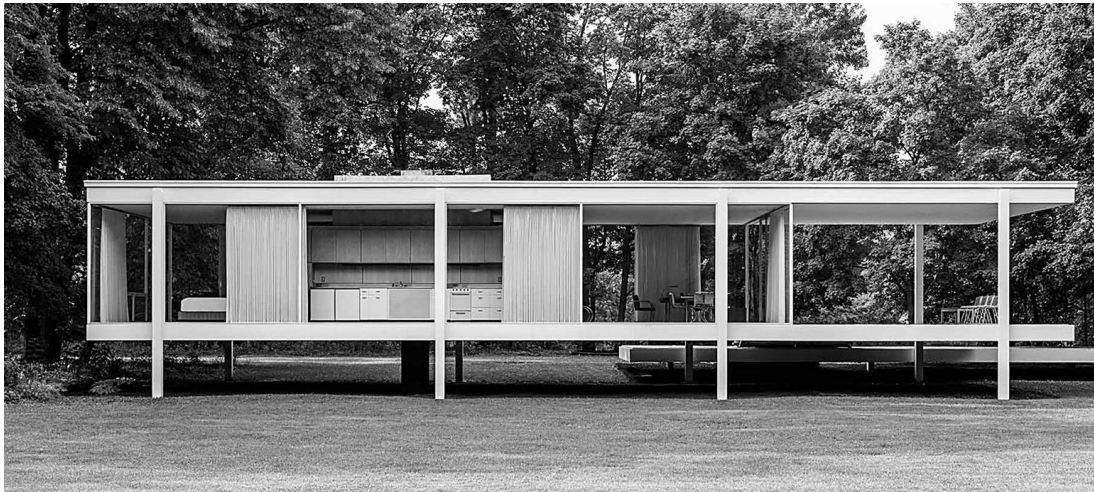
Figure 101. Farnsworth House; A Minimalistic Single-Space Box In Which The Interior Space Is Surrounded Merely By Large Floor-To-Ceiling Glass Window Walls. (Clemence, 2006)
