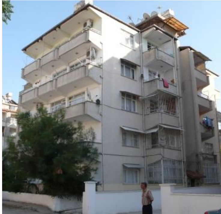
Figure 8: Studied apartment view in Antakya, Turkey
