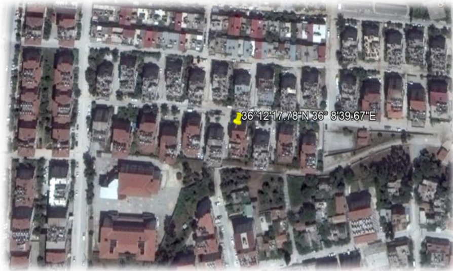
Figure 7: Location of studied apartment in Antakya, Turkey
