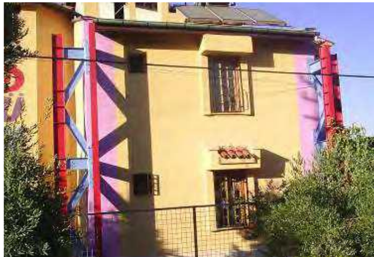
Figure 3: External steel bracing frame out of a structure
