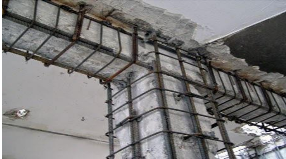
Figure 4: Retrofitting the connection using jacketing by reinforcement concrete, (DEPTA Engineering)
