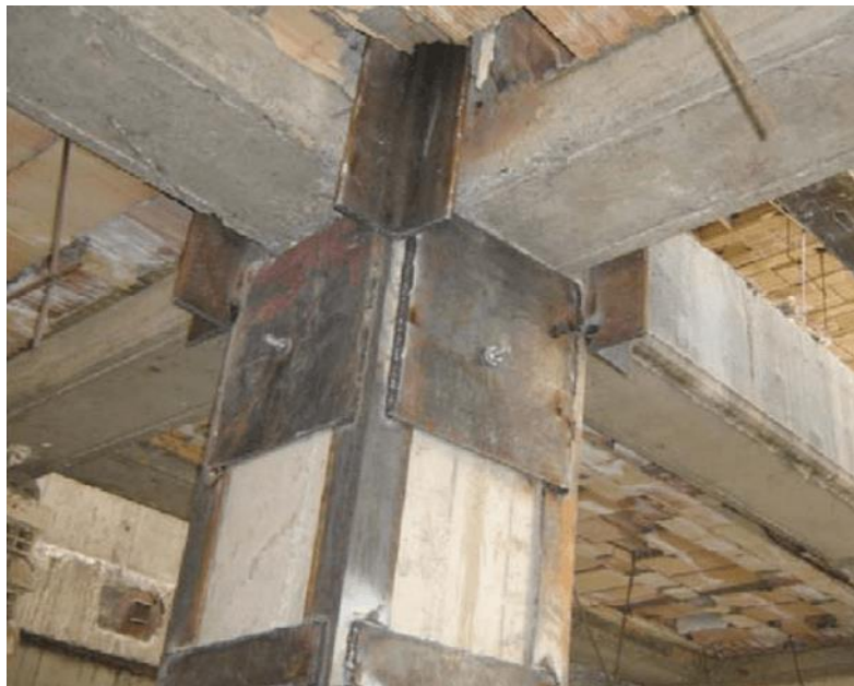
Figure 5: Using steel jacketing for connection (RADYAB Engineering Solution)
