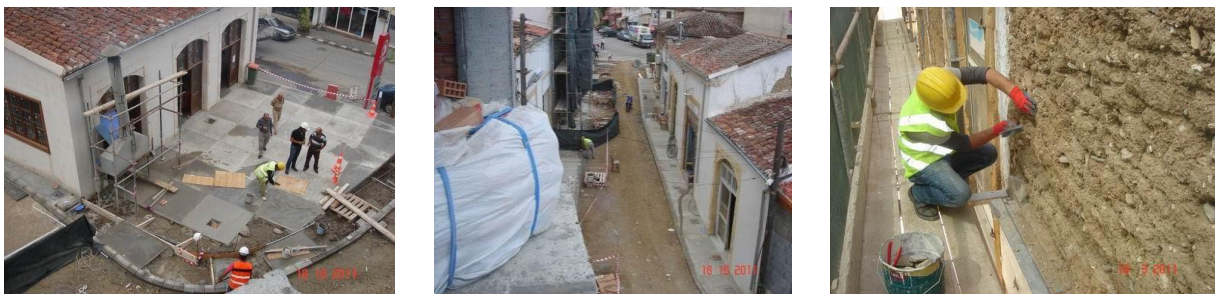
Figure 19: During Improvement in the Area
