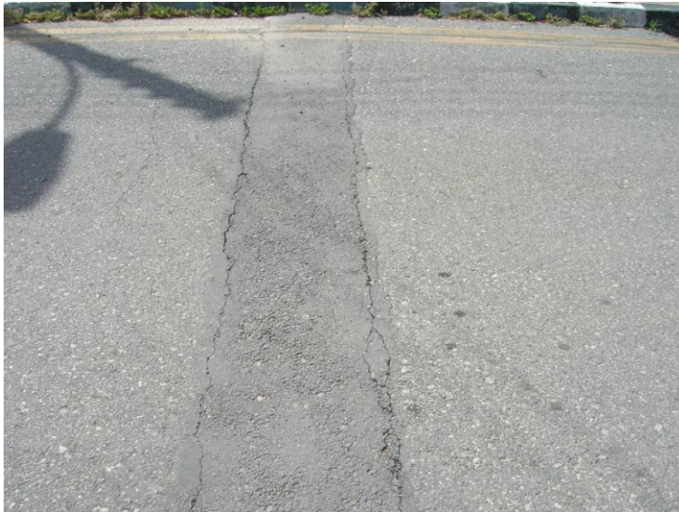
Figure A3. Patching
