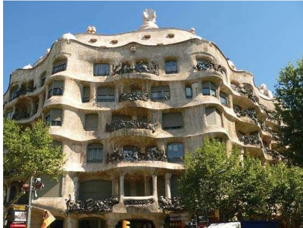
Figure 20: Main façade of Casa Mila, Spain, by Gaudi (britannica, 2019)
