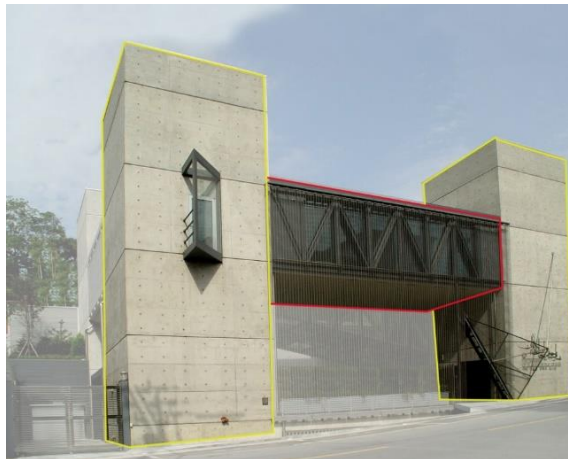
Figure 95: External Analysis of the Embassy. Exposed concrete towers and its connecting exposed steel trusses as semi efficient structure.
