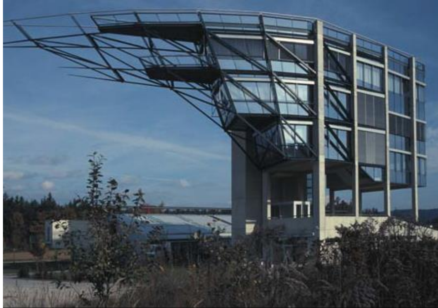
Figure 28: Industrial Park Office Building, Völkermarkt, Carinthia, Austria, Günther Domenig, 1996. The framed block supporting the cantilever and the lift and stair tower behind. (Charleson, 2005, p. 205)
