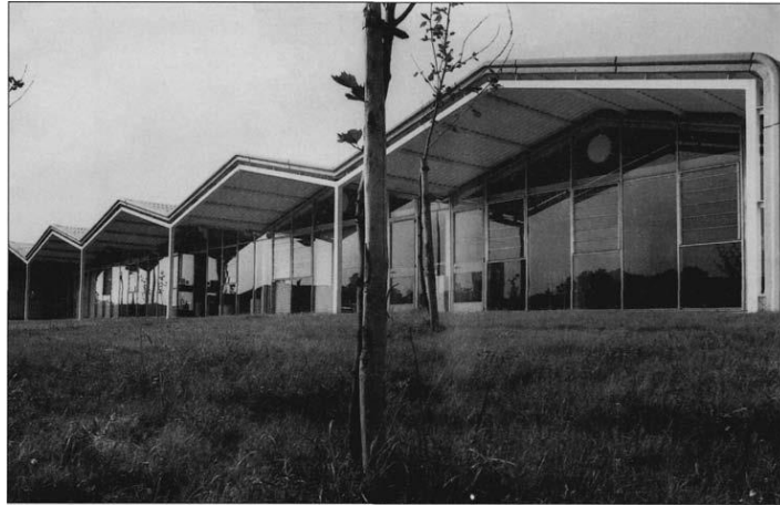
Figure 128: Palmerston Special School, Liverpool, England 1973-76 (demolished 1989). Foster Associates, architects; Anthony Hunt Associates, structural engineers. Semi-formactive portal frames of steel hollow-section are used here as the primary structural elements in a multi-bay arrangement with relatively short spans. The moderately high efficiency of this type of structure has permitted very slender elements to be adopted. (Macdonald, Structural Design for Architecture , 1997, p. 12)
