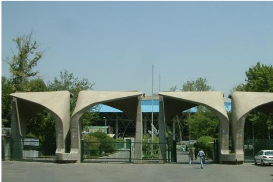
Figure 36: Main designed gate of University of Tehran, Iran
