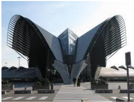
Figure 19: Façade of the Lyon airport railway station (structurae, 2016)
