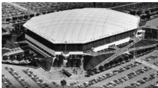
Figure 127: Barton Malow Silverdome. A very large span is achieved here with a cable-reinforced air-supported membrane, which is a tensile form-active structure. (Macdonald, Structure and Architecture, 1994, p. 58)
