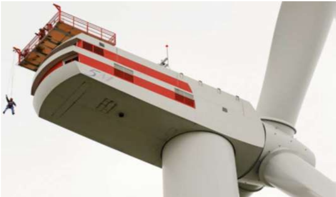
Figure 2.15: a) Installation technique by using one vessel in long distance OWFs, and b) Close shot of nacelle of a 5MW offshore WT
