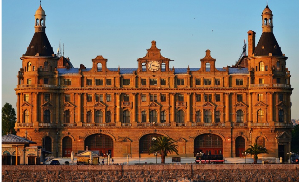
Figure 57: Haydarpaşa Train Station Facade (URL50)
