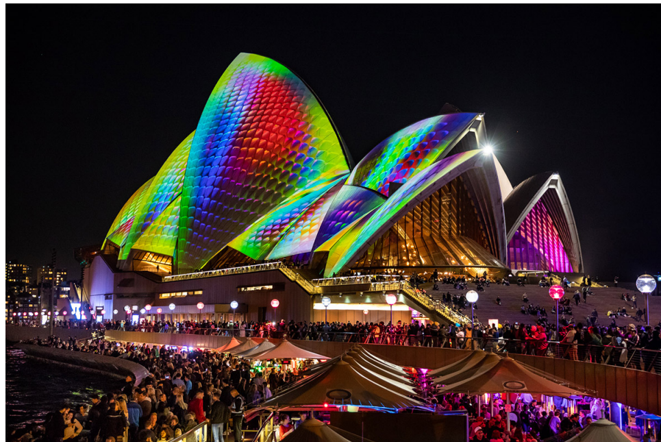
Figure 43: Sydney Opera House Illuminated, Project Vivid (URL43)
