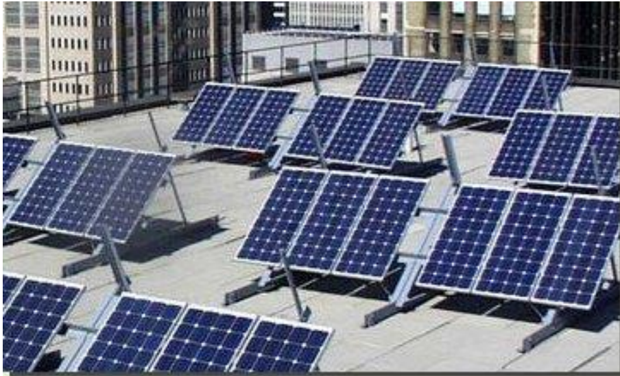
Figure 3.5. Free standing PV on roof ( http://www.greenbuildingenergysavings.com )
