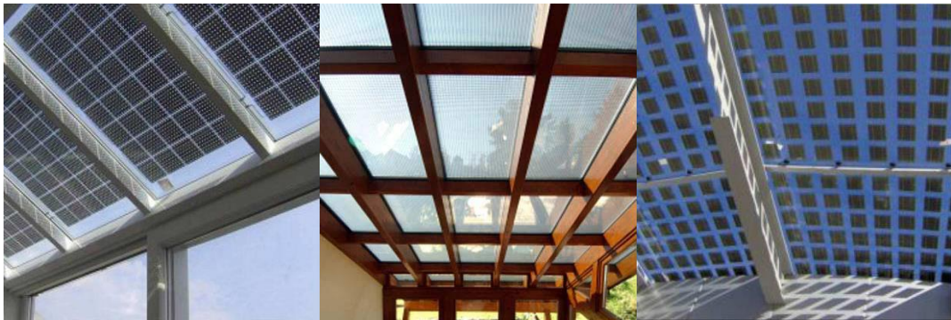
Figure 2.6. Examples of Translucent Panels ( http://www.bipv.ch/index.php/en/visual-aspects/frame-color )
