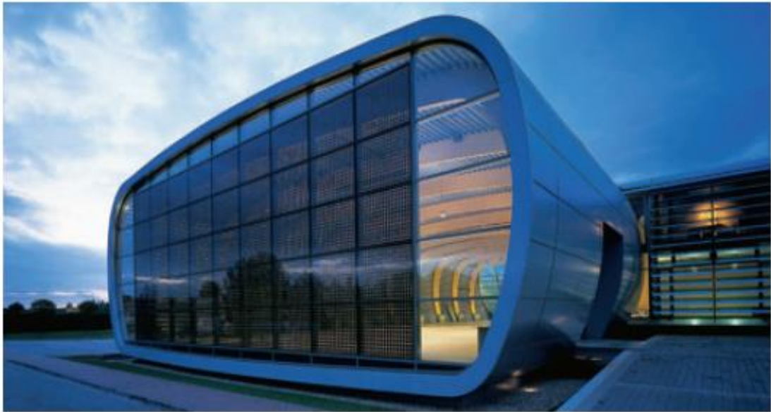
Figure 3.10. Example of a structural sealant glazing facade with PV modules in the form of insulating glass units (Pierre, 2003)
