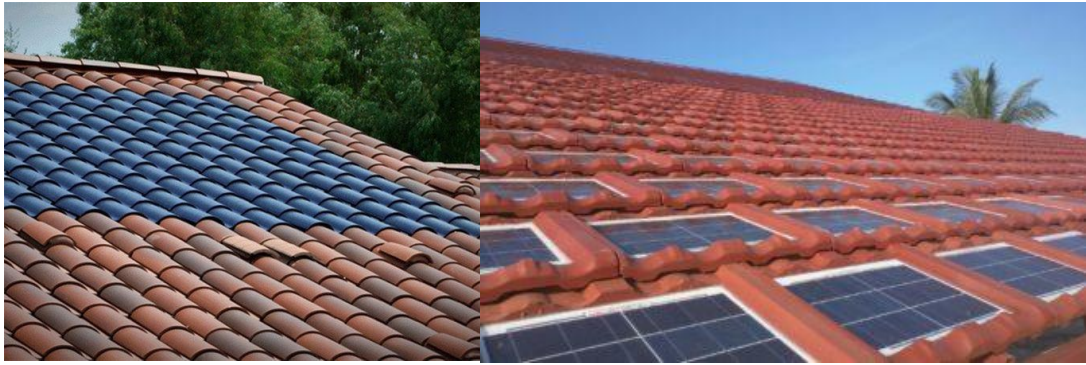
Figure 2.10. Roof and translucent glazing integration examples (Jelle, 2012)
