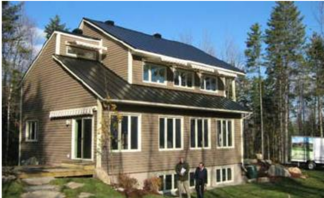
Figure 4.4. The Eco Terra house in Eastman, Canada (Noguchi et al., 2008)
