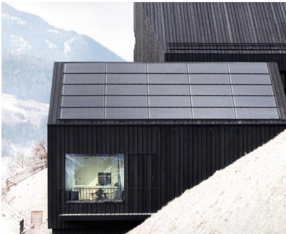
Figure 4.5. La Pedevilla Chalet BIPV roofing system (Maturi and Adami, 2018)
