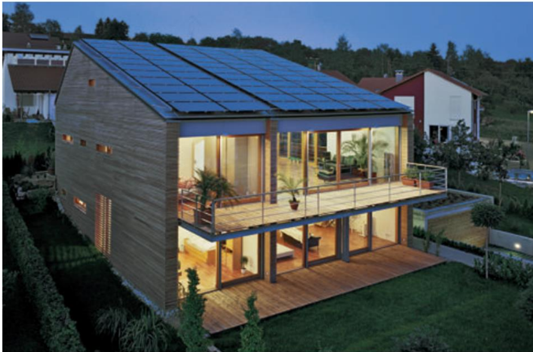
Figure 4.3. The Private house in Hegenlohe with PV integration (Maturi and Adami, 2018)
