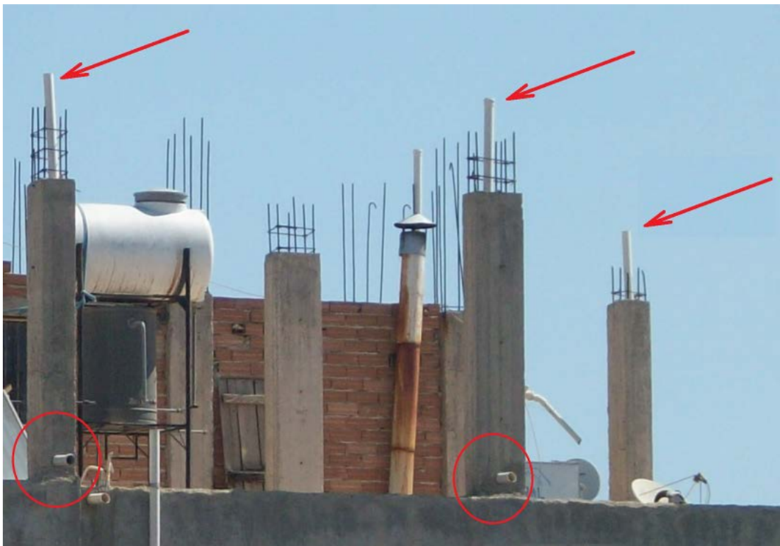
Figure 1.2. Pipe embedded in RC columns
