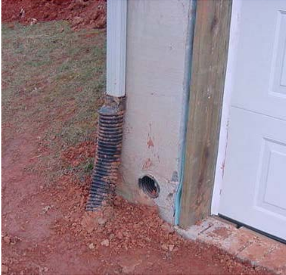
Figure 1.3. Pipe exit at ground floor
