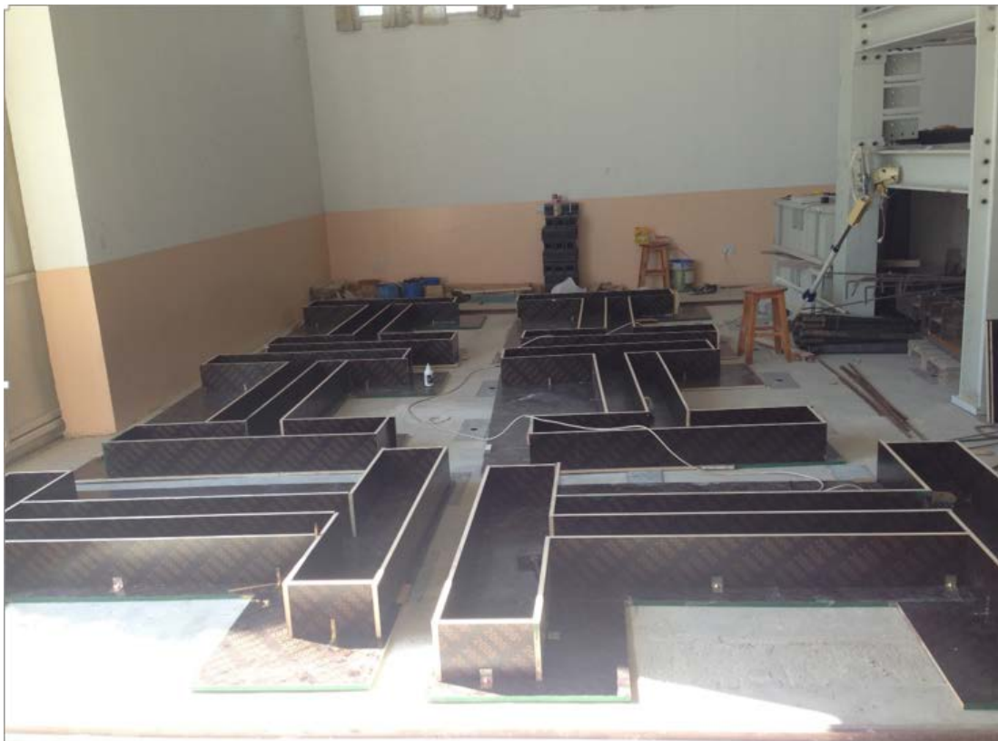
Figure 3.5. Prepared formworks before reinforcement placement
