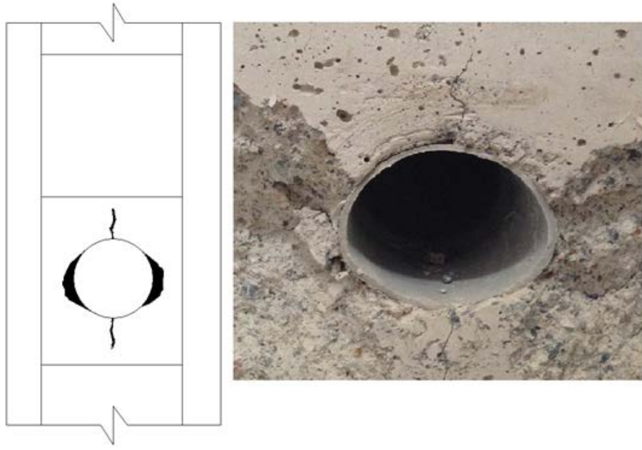
Figure 5.4. State of specimen C-1 after the test
