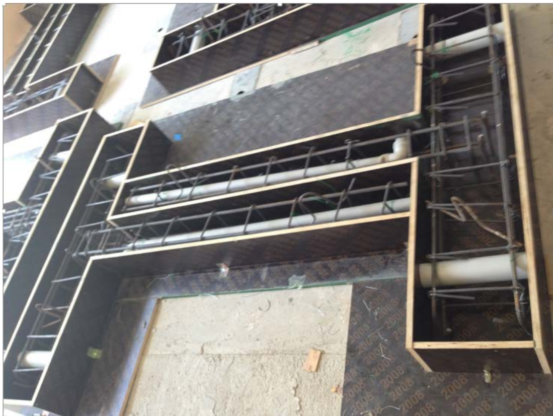
Figure 3.9. Placement of reinforcements and PVC pipes in formwork
