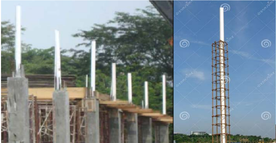
Figure 1.1. PVC pipes embedded in columns
