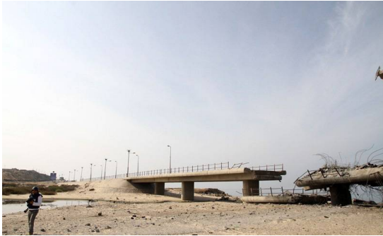
Figure 38: Destroyed Bridge, Photo Retrieved from (URL24)
