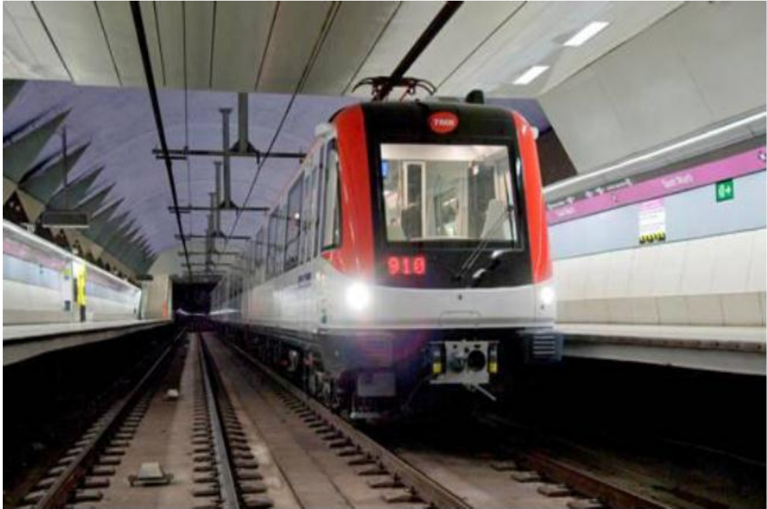
Figure 3: Barcelona Metro Line 9 (Fuente et al., 2014)
