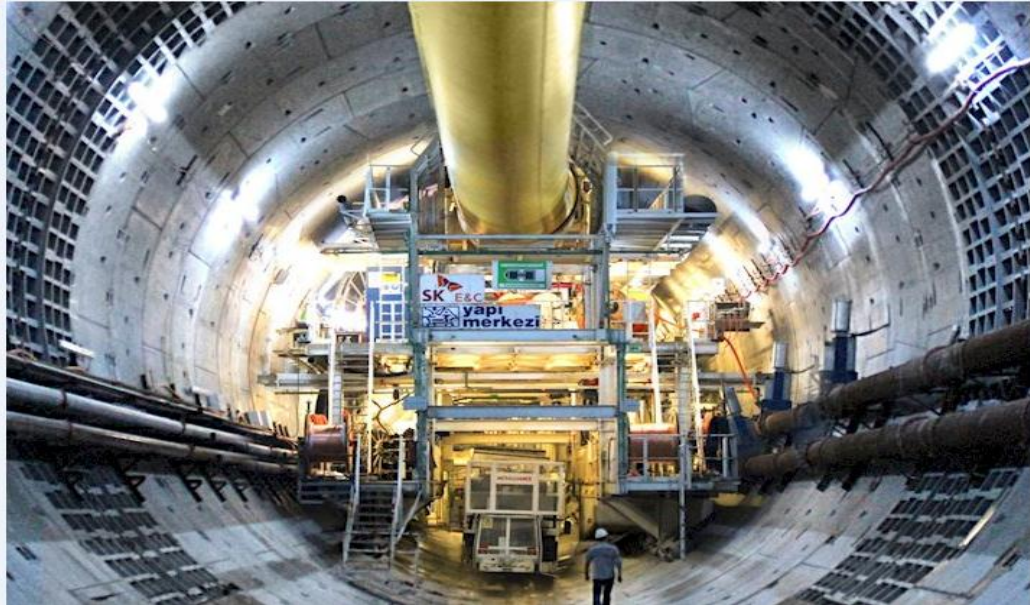
Figure 4: Eurasia Tunnel in Turkey (Istanbul Metropolitan Municipality, 2016)
