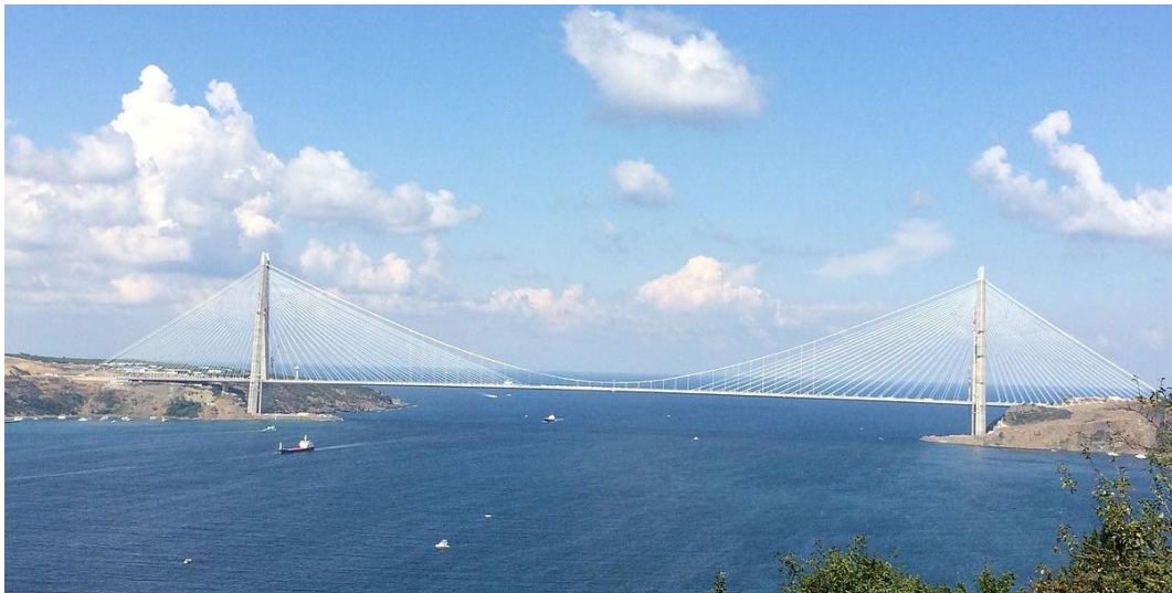
Figure 5: Yavuz Sultan Selim Bridge in Turkey (Istanbul Metropolitan Municipality, 2016)
