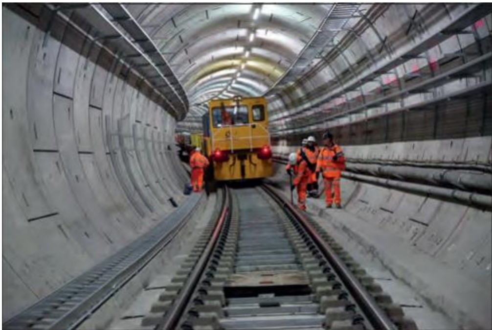
Figure 2: Rail System installation of Elizabeth line in the UK (Tucker, 2016)
