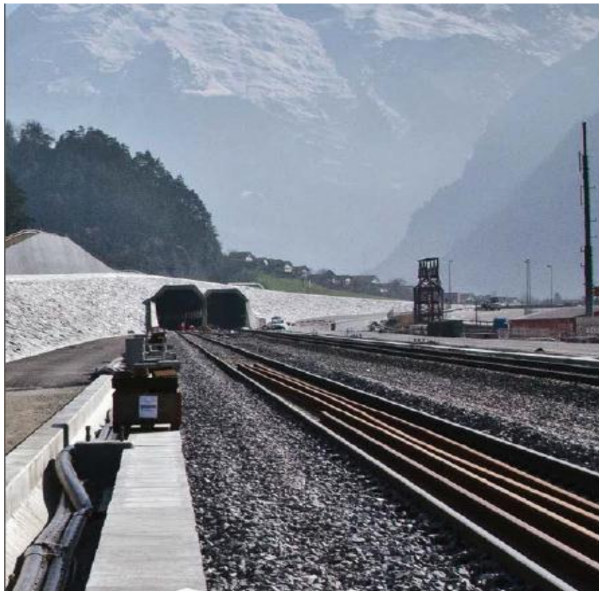
Figure 1: Gotthard Base Tunnel through Alps in Switzerland (Alptransit, 2016)
