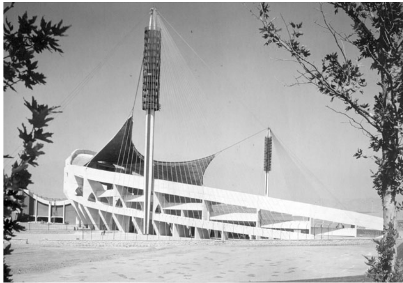
Figure 12: Shiroodi (former Amjadieh) Sports complex (1973). Architect: Jahangir Darvish. http://www.caoi.ir/en/projects/item/283-takhti-stadium.html
