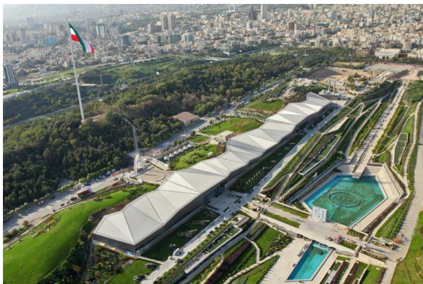
Figure 22: Holy Defense Museum, Tehran (2010). An example of the contemporary attempt in the design of public buildings in Iran.
