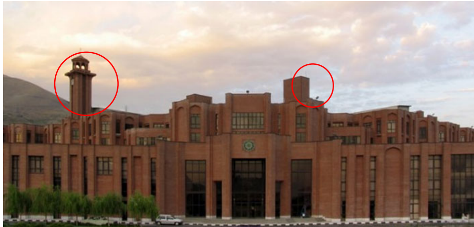
Figure 77: a general view on the main façade of the project. http://raahak.com/?p=9027
