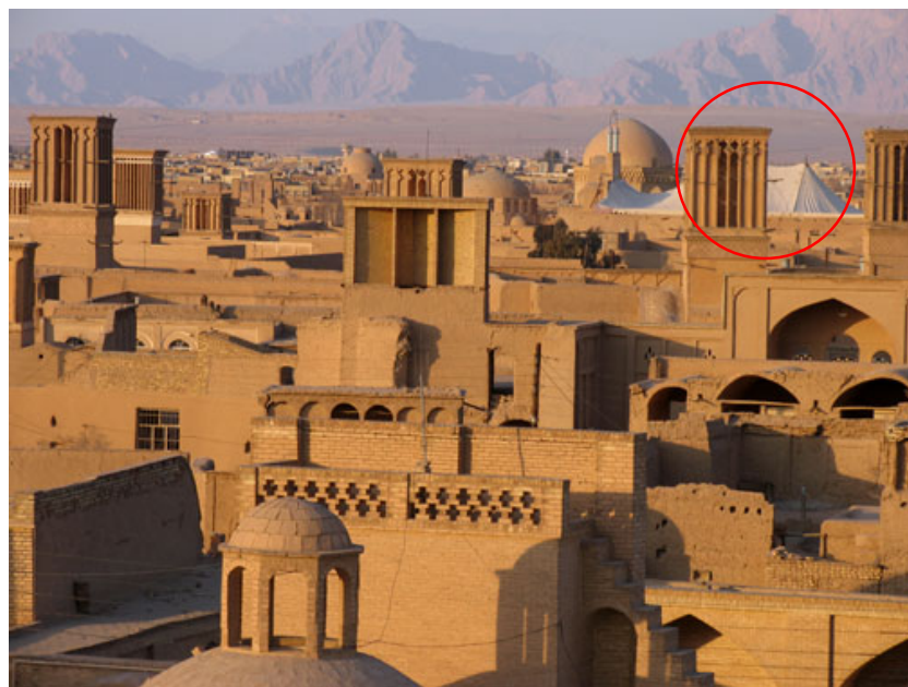
Figure 78: density in the urban context of Yazd, a city in the hot and arid climate of Iran. Wind catcher is an important element in this climate. https://www.wipolo.com/en/destination/1146320/yazd.html
