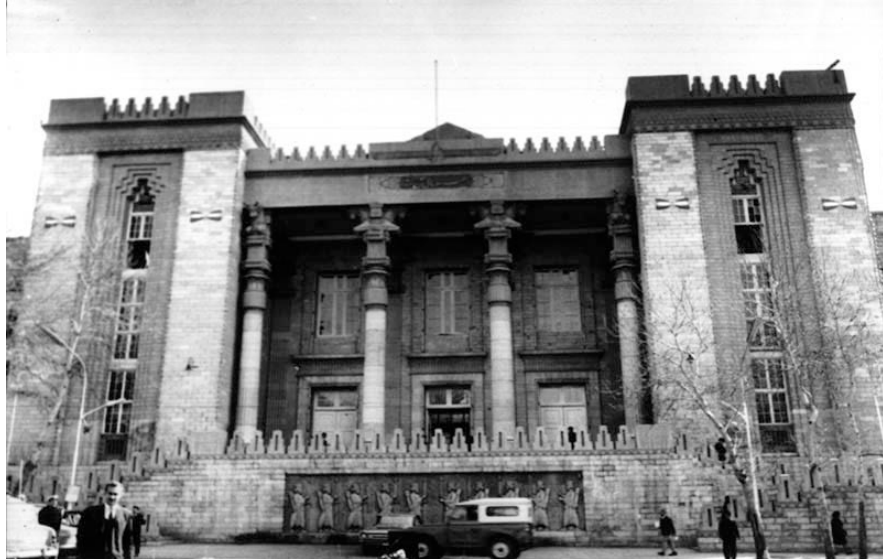
Figure 38: Police head Quarters (1937), Main entrance. Tehran. Architect: Mirza Alikhan Mohandes. http://1host2u.com/?ez=6502
