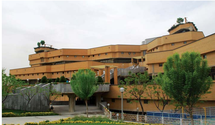
Figure 68: Brick and Stone on the façade of the National Library https://safarzon.com/mag/
