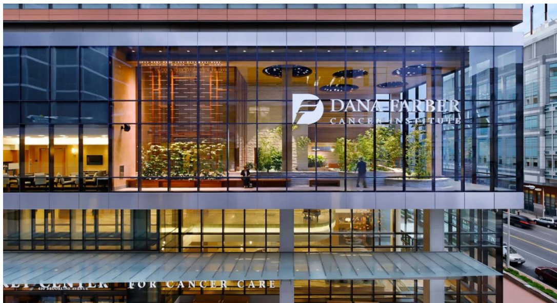
Figure 14: The exterior view of the garden serves as a beacon and a symbol of healing. The garden's third-floor location and lush plantings afford privacy for garden users (URL 7).
