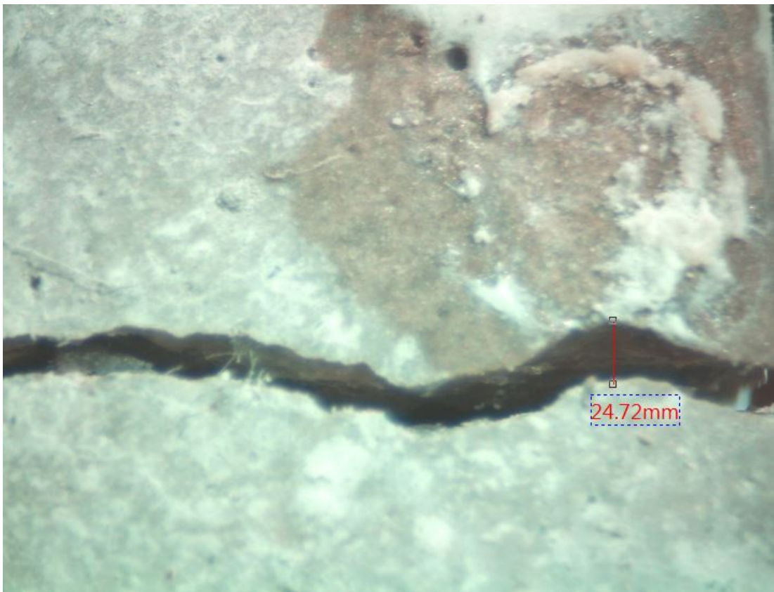
Figure 46c: HSC-20% PP surfaces after 200 °C heating at 28 days
