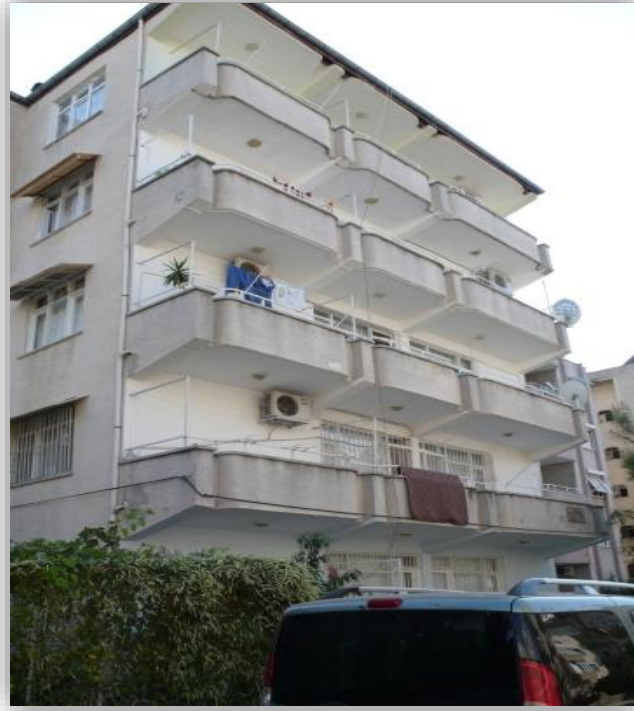
Figure 3.3: Studied apartment view in Antakya, Turkey.
