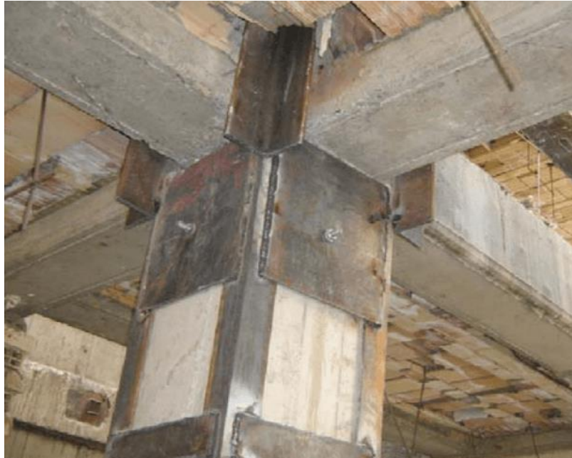
Figure 2.5: Using steel jacketing for connection (Source: RADYAB Engineering Solution).
