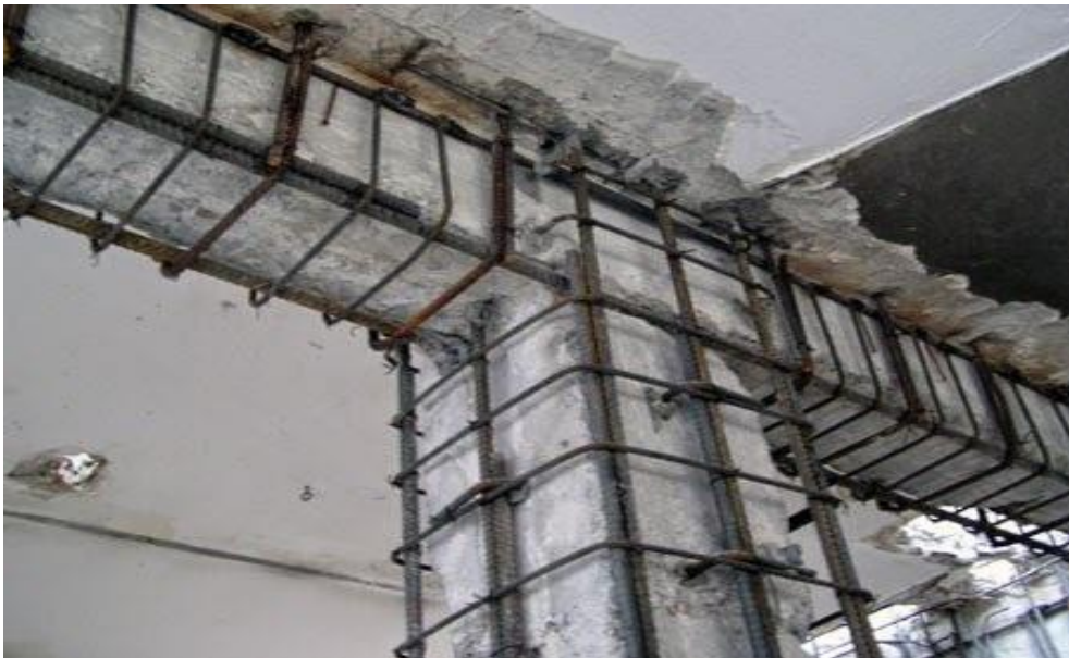
Figure 2.4: Reinforced concrete jacketing (source: DEPTA Engineering).
