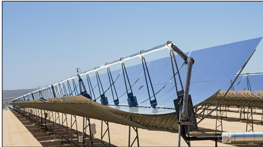
Figure 6: Cylinder-Parabolic Solar Collector
