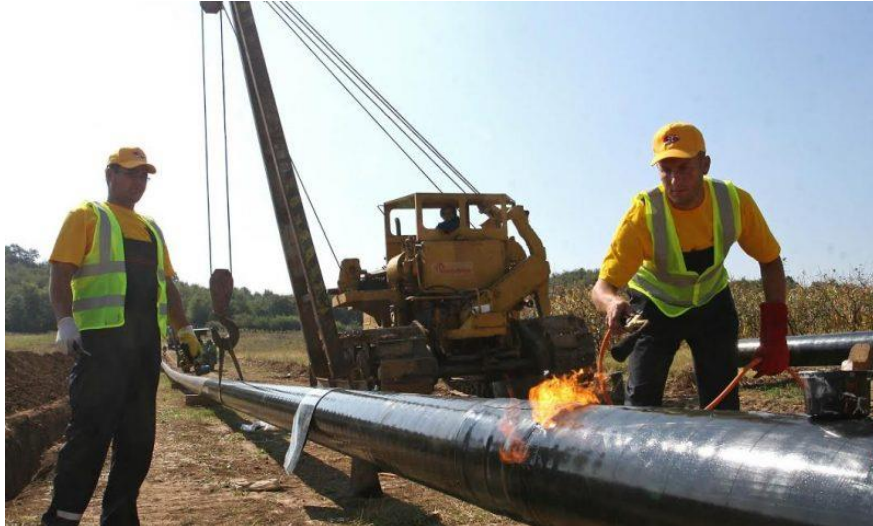
Figure 3.4: The procedure of the pipeline installment onshore
