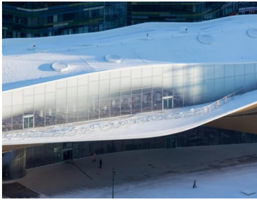
Figure 62: Cantilevered library balcony; (URL 66)
