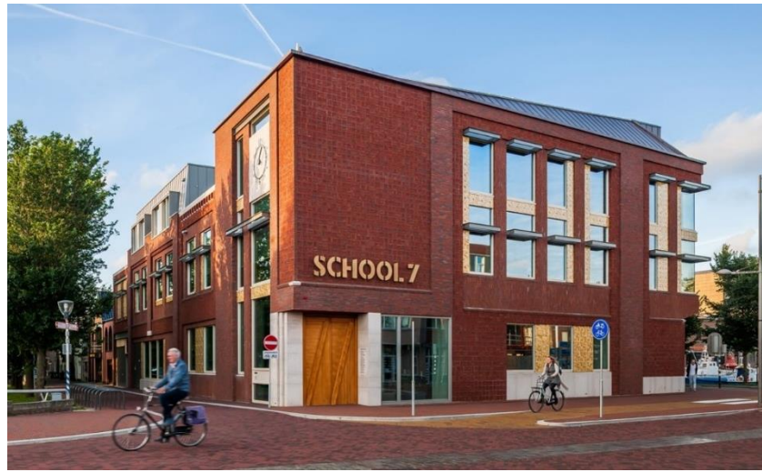
Figure 65: School 7 exterior view; (URL 69)
