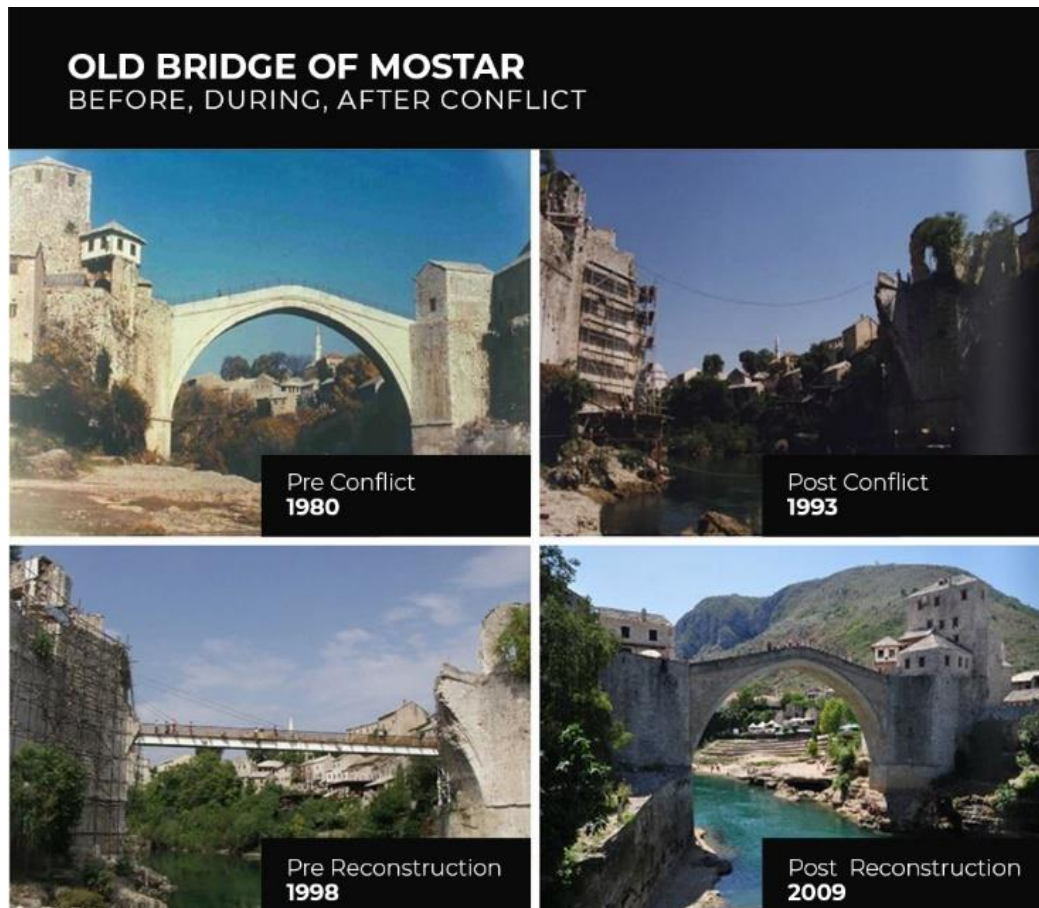
Figure 4.12: Old Bridge of Mostar Before, during and After Conflict (adapted from UNESCO, 2021; URL24; URL25; URL26; URL27)
