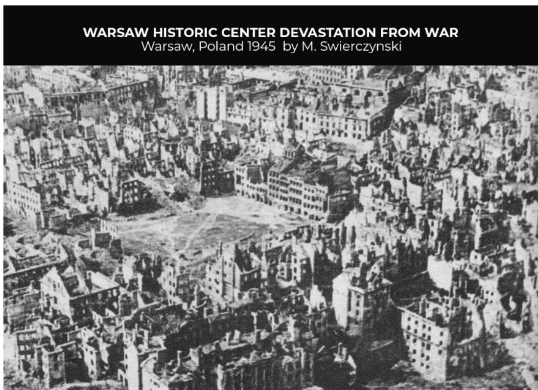
Figure 4.20: Aerial picture of Warsaw, Poland, demonstrating the devastation caused by the war and a recent revolt, January 1945 (Photo: M. Swierczynski, URL29)
