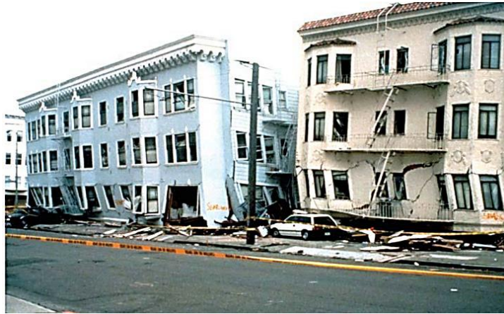
Figure 6: Collapse and deformation of structures in the Loma Prieta earthquake [18]
