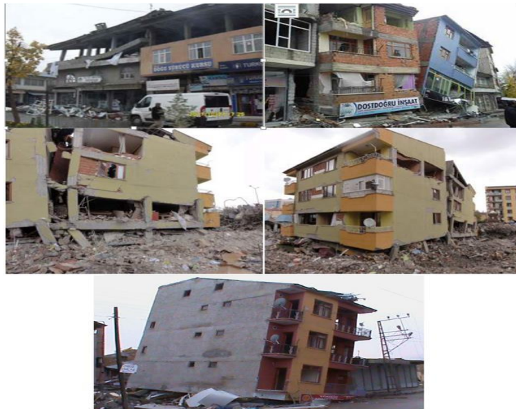
Figure 10: Occurrence of soft story in 2011 Van Turkey earthquake[18]
