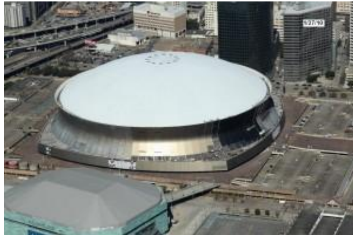
Figure 72: Lamella Dome (Schueller, 1996)
