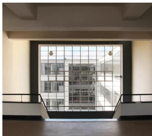
Figure 8: Dessau Bauhaus interior view (URL2)
