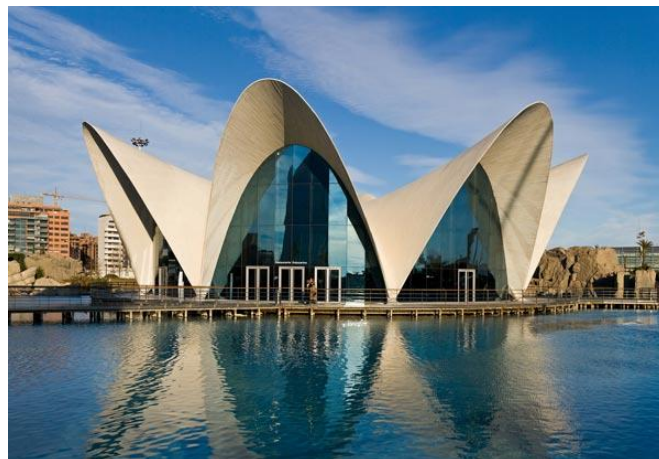
Figure 74: Example on hyperboloids of revolution, shell structure (URL25)
