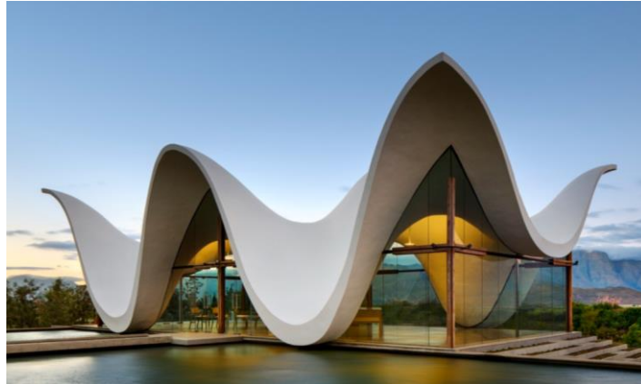
Figure 73: Example on concrete shell structure (URL24)
