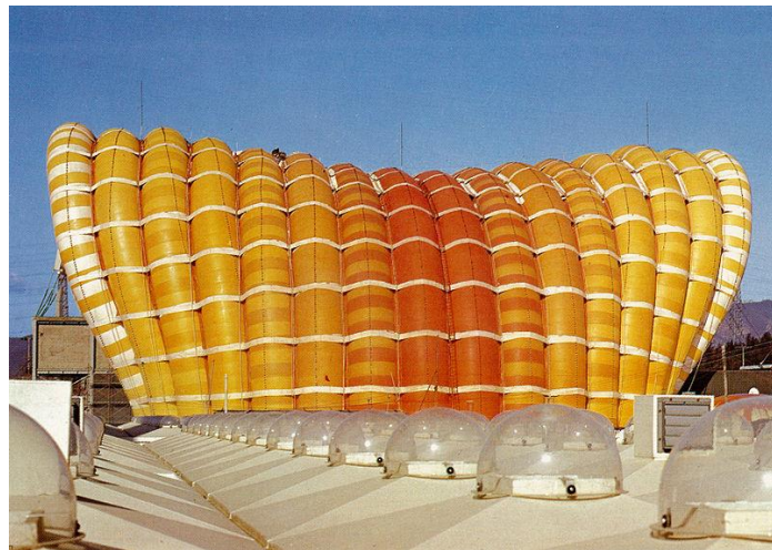
Figure 75: Example on Pneumatic structure, exhibitions reached a peak the EXPO'70 in Osaka (URL266)
