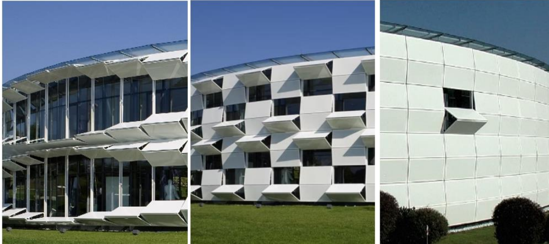
Figure 16: Shown the Responsive Façade the on Left When It Fully Open, on the Middle Semi Closed and, on the Right, Fully Closed. Kefir Technic Showroom, Badgley Chenberg, Austria, URL9.
