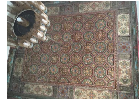
Figure229: ceiling in the hall (by author, 2019).
