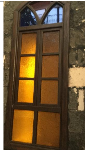
Figure231:Interior window (by author, 2019).
