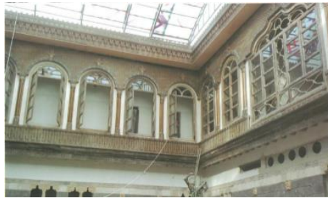
Figure 28:Interior windows on the first floor. (Amene, 2018)
