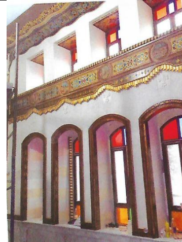
Figure245: Interior windows in first floor (by author, 2019).
