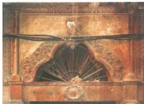
Figure 27: The upper openings of the external doors. (Amene, 2018)
