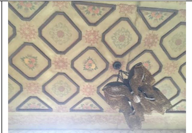
Figure212 : Ceiling in the room (by author, 2019).
