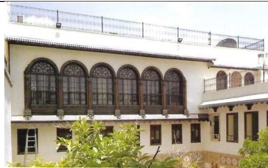
Figure248: interior windows first floor (by author ,2019).
