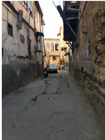
Figure 9: The exterior facades in old Damascus (by author).
