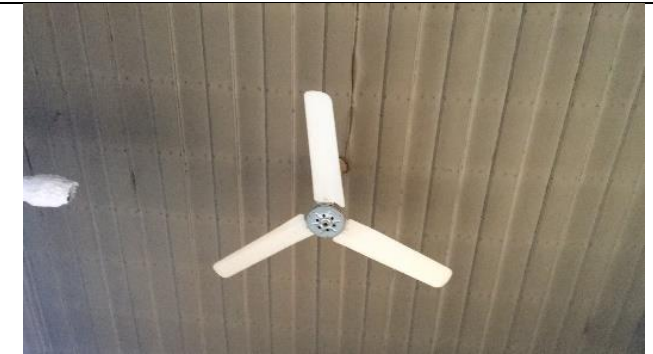
Figure141: :Ceiling of the bedroom in the first floor (by author, 2019).
