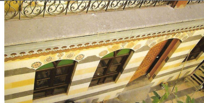
Figure215 : Interior windows (by author, 2019).
