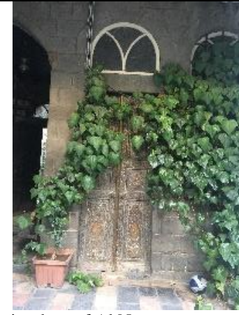
Figure108: interior door of Al Nasaane courtyard house ( by the athor2019).
