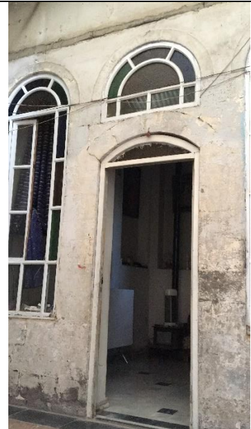
Figure142: interior door in the courtyard (by author, 2019).
