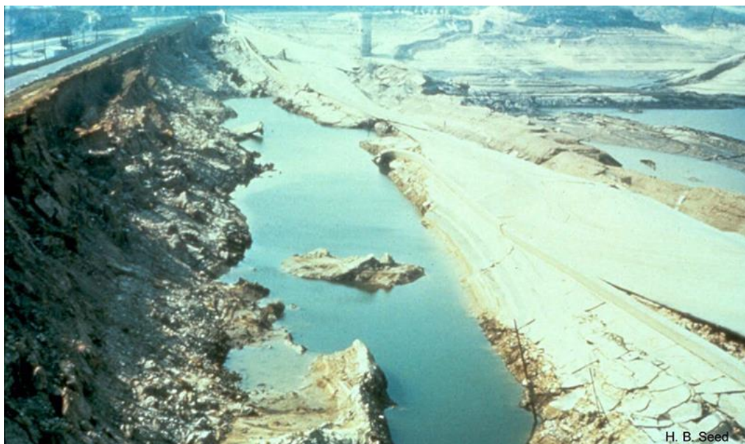
Figure 1: Upstream face San Fernando Dam flow liquefaction (Geo-Slope International Limited).
