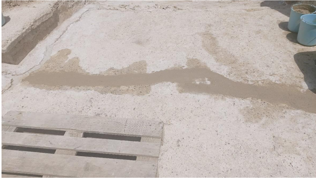
Figure 2.10: Repaired cracks at roof
