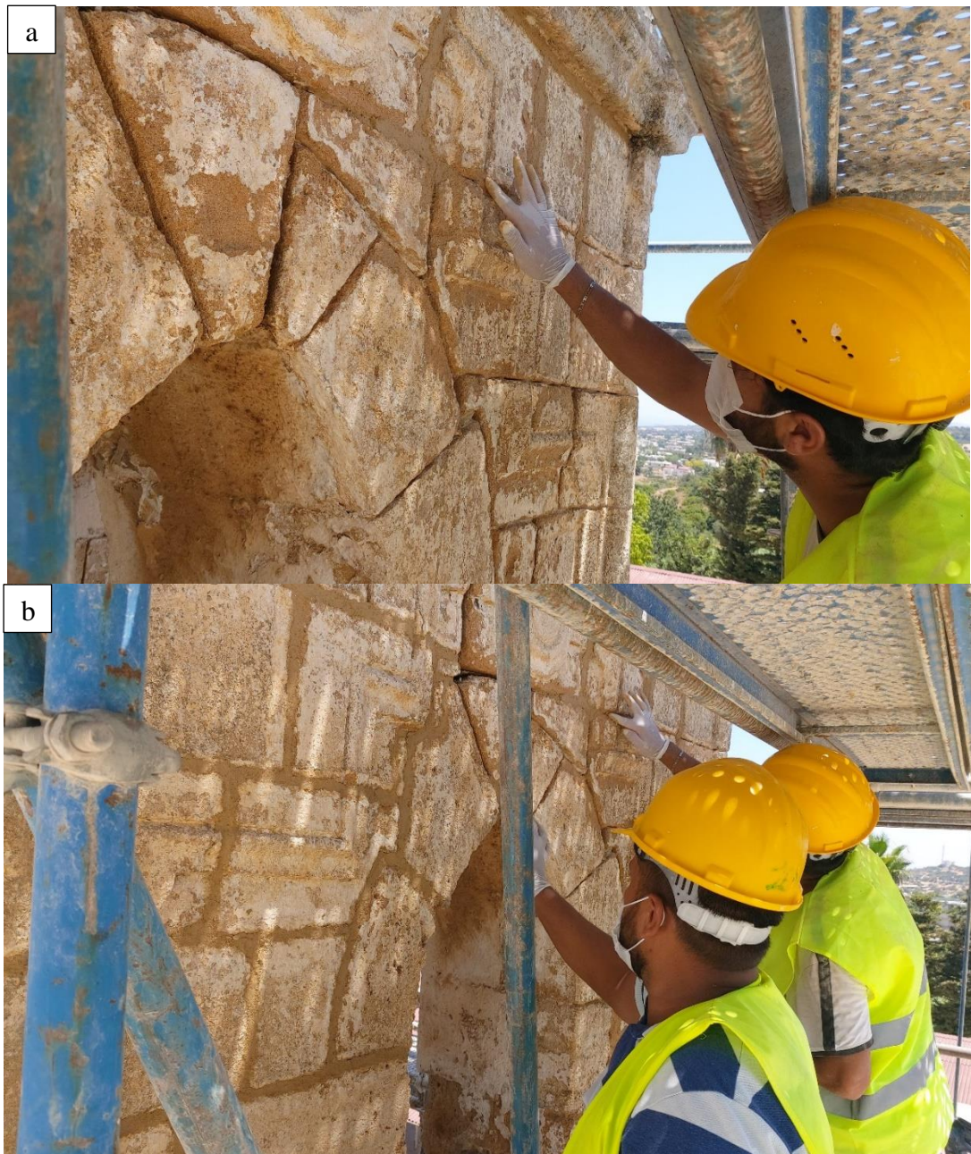
Figure 2.42: a) Repointing of belfry 1 b) Repointing of belfry 2
