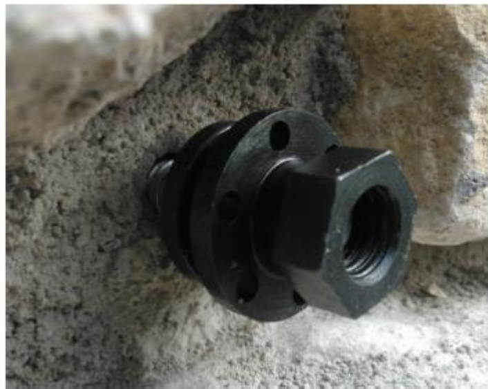
Figure 2.70: Cord locking device inside the wall joint before application of steel cords and mortar [25]
