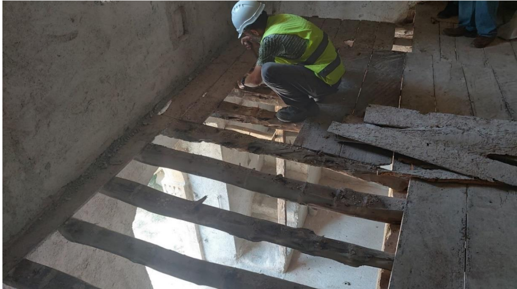
Figure 2.46: Removal of existing substructure floor
