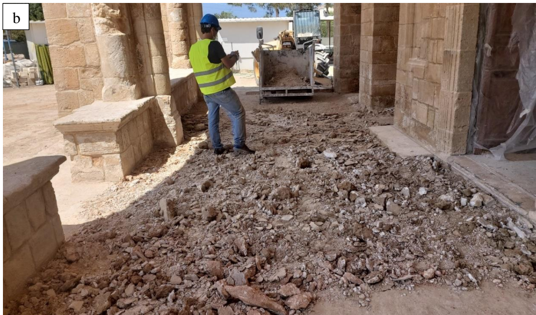
Figure 2.44: a) Removal of existing floor stage 1 b) Stage 2
