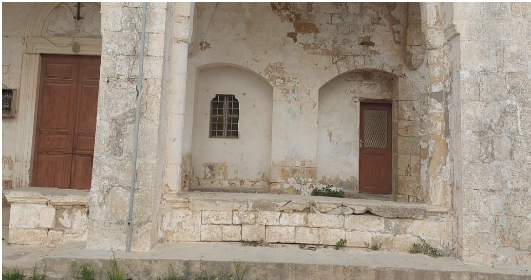
Figure 2.20: Existing cornice stones
