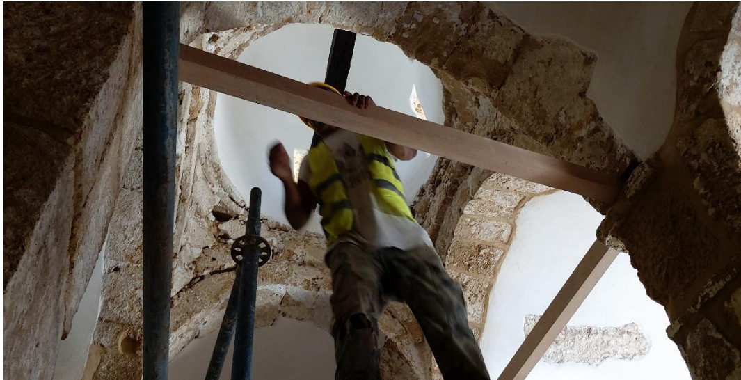
Figure 2.18: New wooden tie beams
