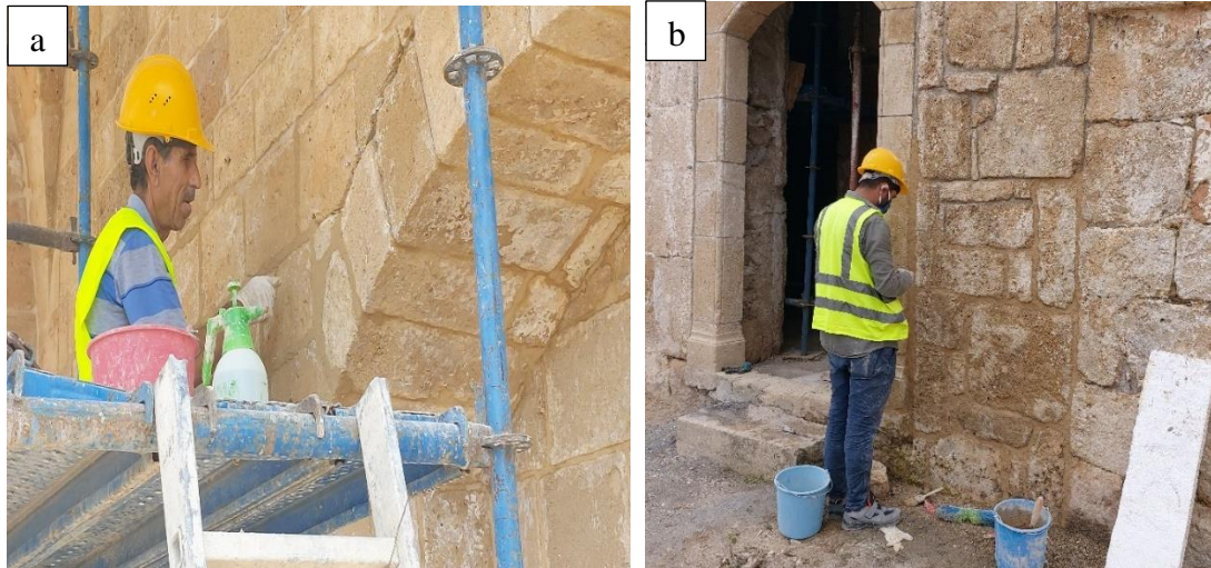
Figure 2.7: a) Repointing 1 b) Repointing 2
