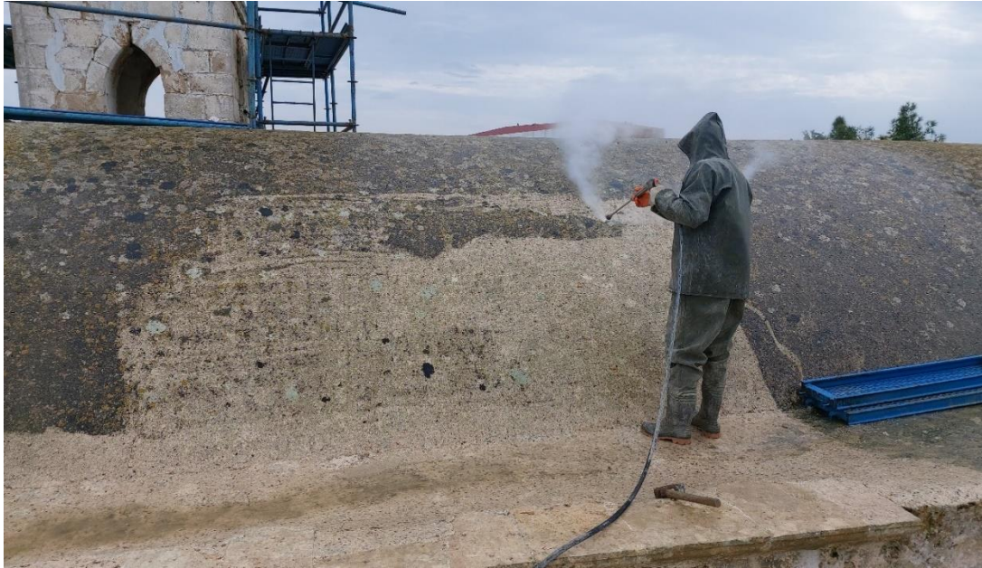
Figure 2.29: Cleaning of loose deposits stage 2
