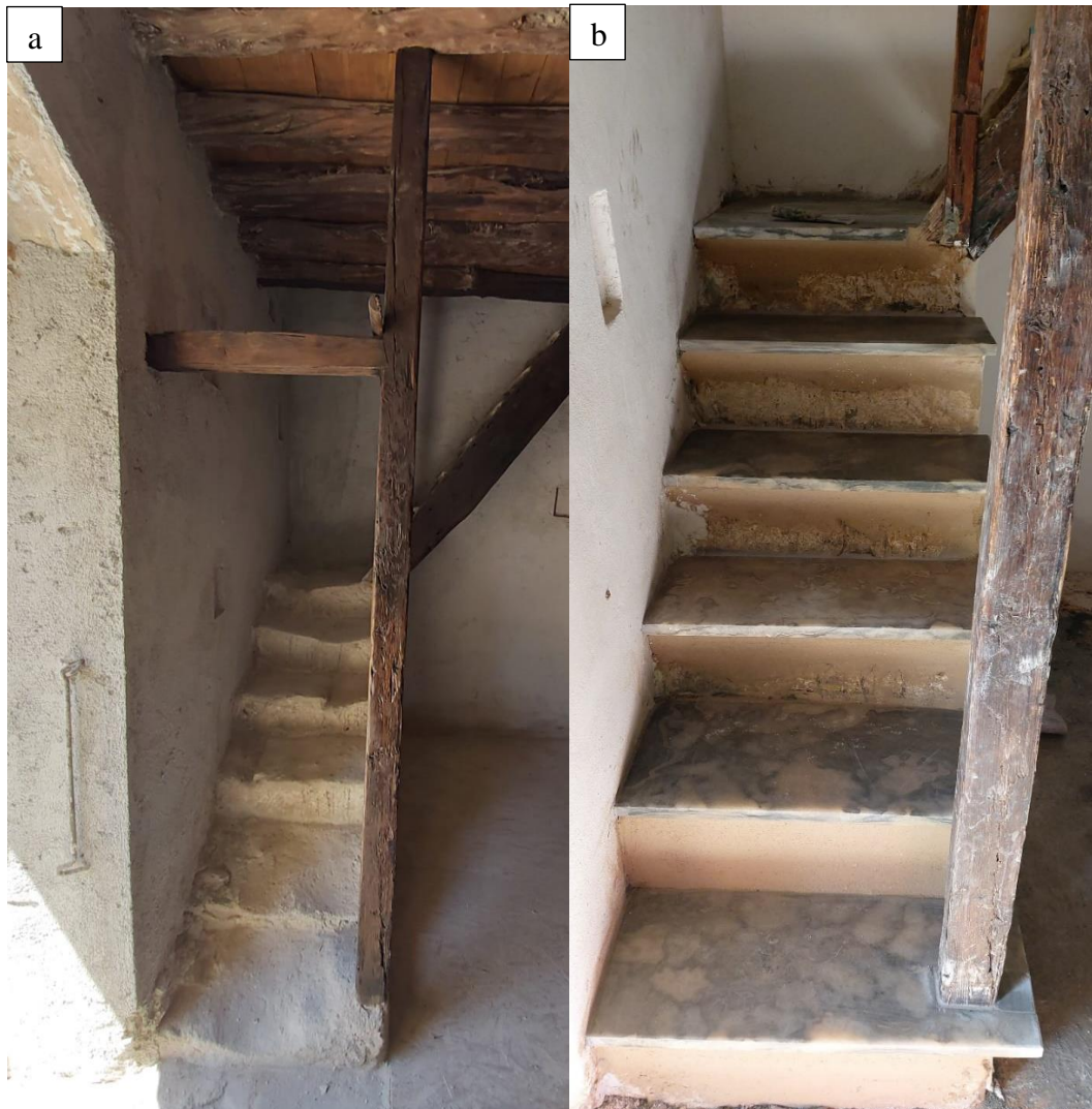
Figure 2.52: a) Initial condition of stairs b) Final condition of stairs
