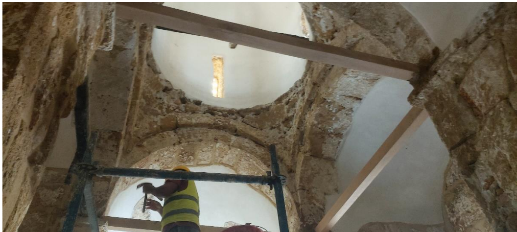
Figure 2.19: New wooden tie beams
