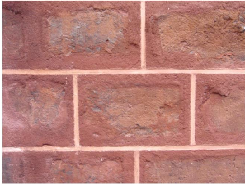
Figure 2.68: Mortar repair of degraded bricks [24]
