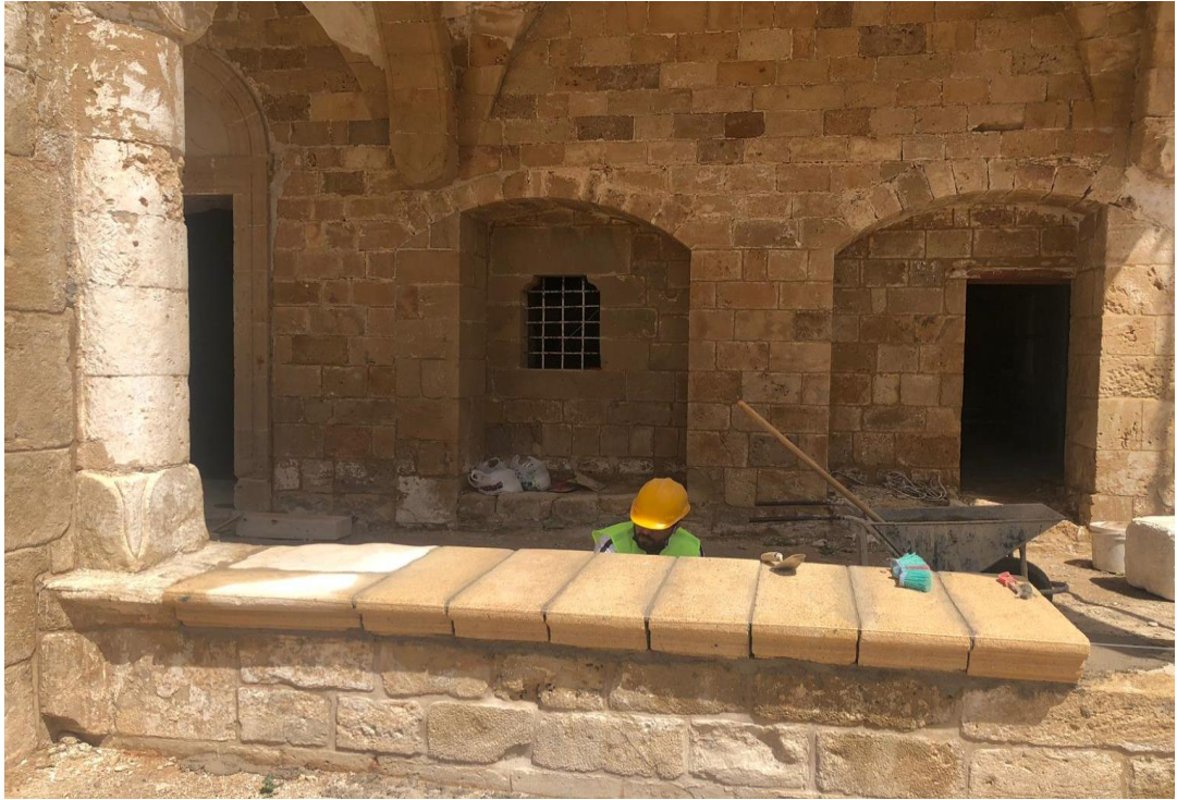
Figure 2.21 New cornice stones
