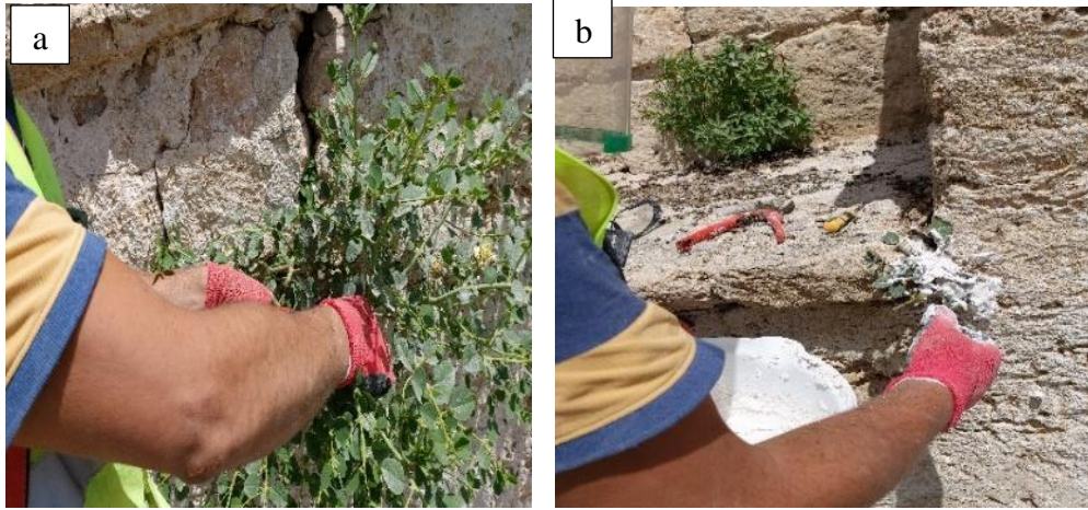
Figure 2.5: a) Vegetation removal stage 1 b) Stage 2
