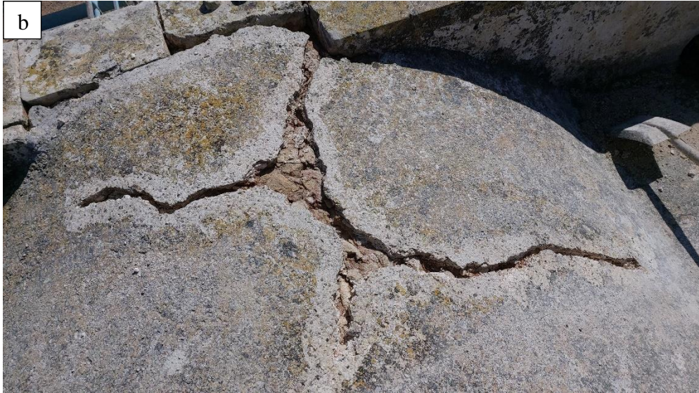
Figure 2.32: a) Removed lime mortar up to a depth of 15 cm 1 b) Removed mortar up to depth of 15 cm 2
