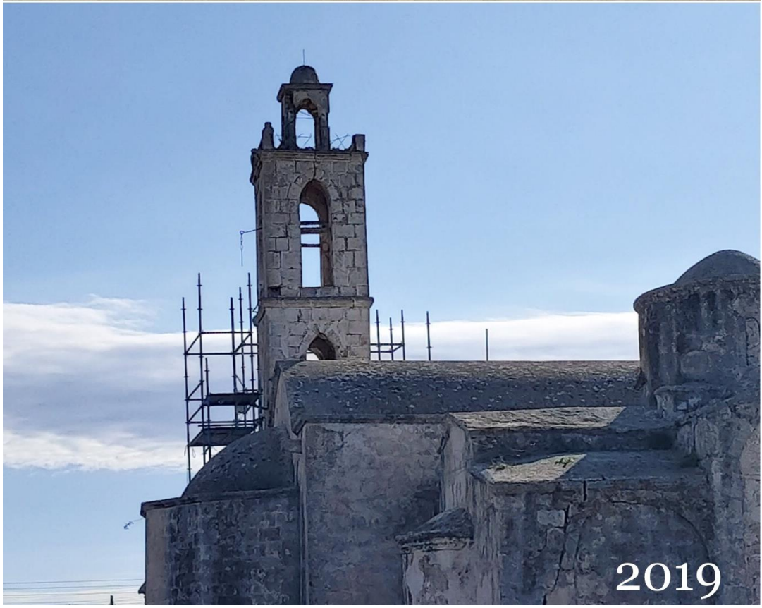
Figure 2.62: View of the roof from northern facade
