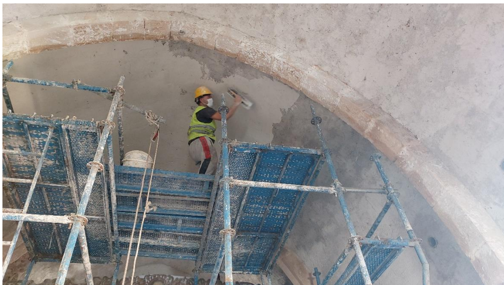
Figure 2.15: Plastering stage 2
