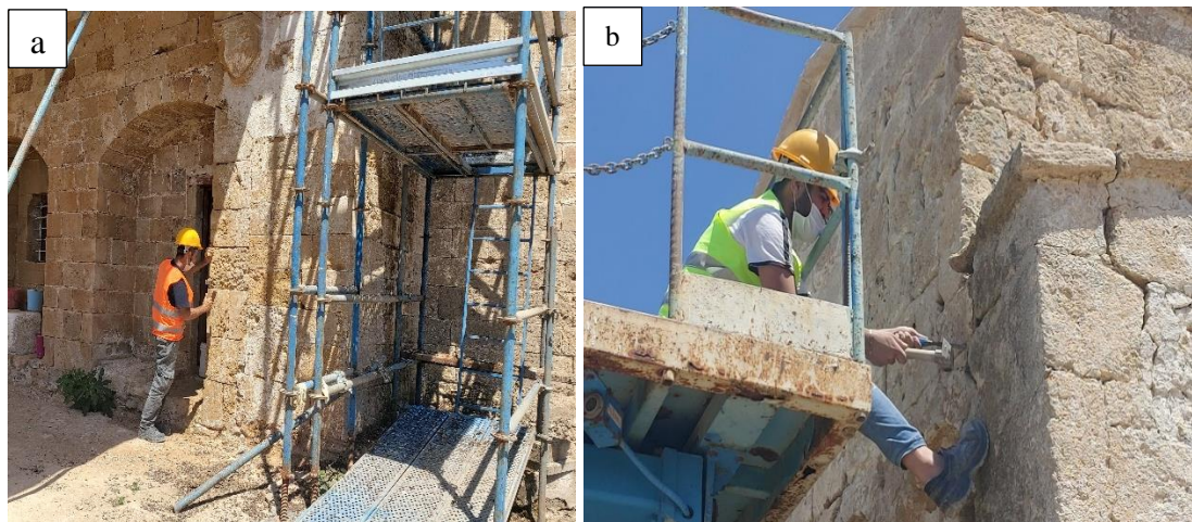
Figure 2.6: a) Pointing removal 1 b) Pointing removal 2
