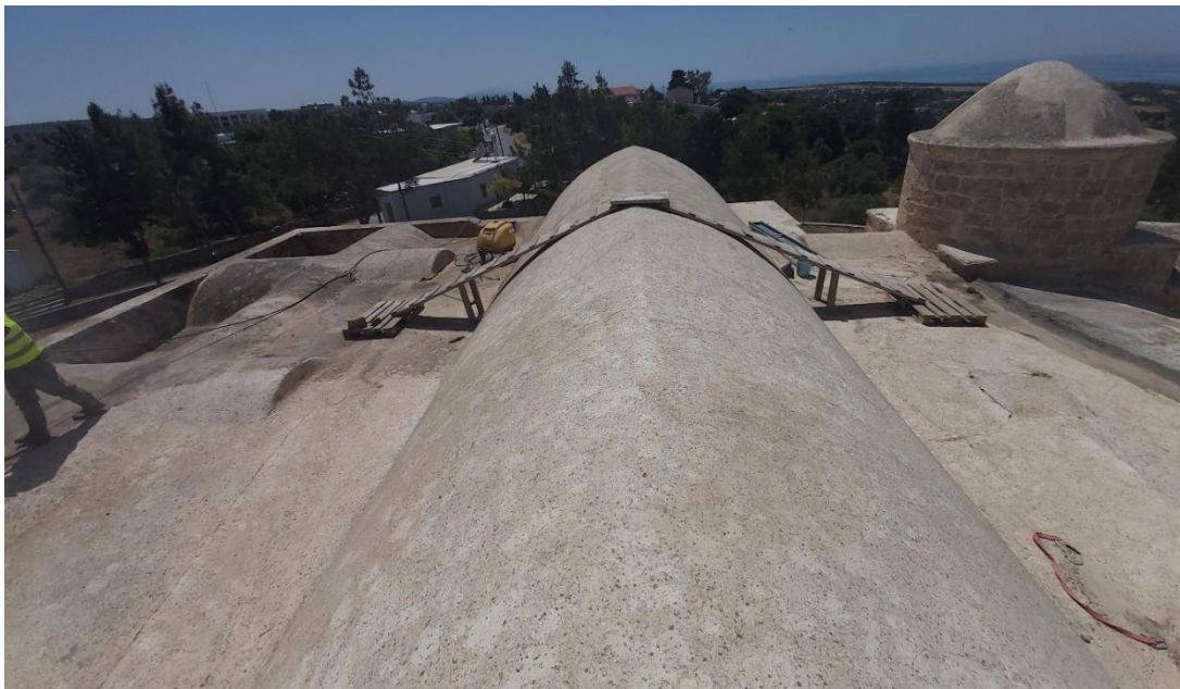
Figure 2.30: Cleaning of loose deposits stage 3
