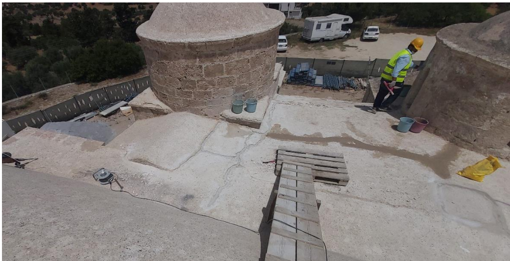
Figure 2.11: Repaired cracks at roof
