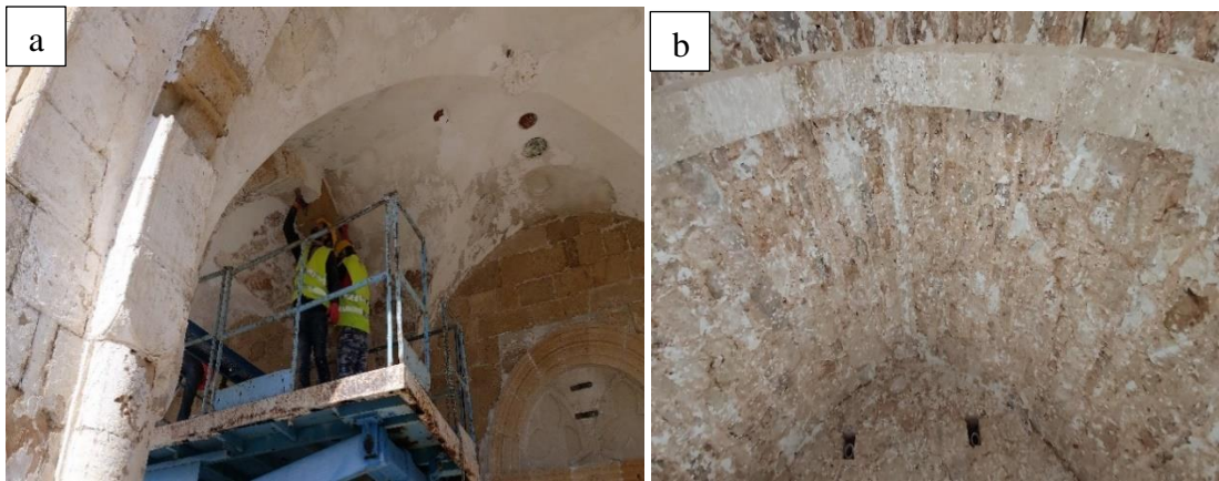
Figure 2.12: a) Initial condition b) After of cement removal
