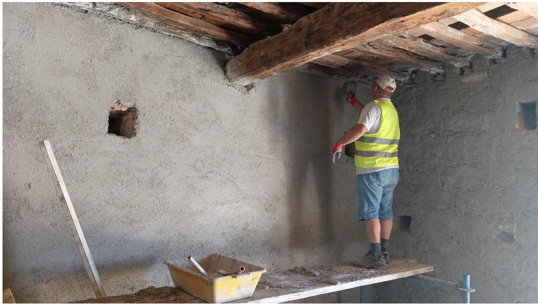
Figure 2.14: Plastering stage 1
