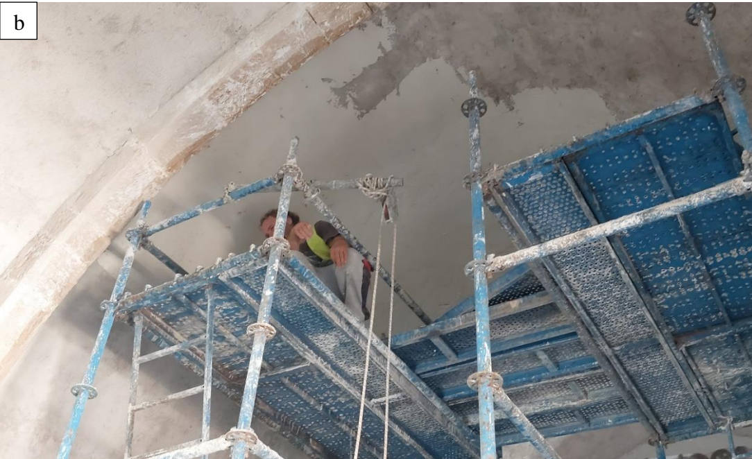
Figure 2.26: a) Plastering of ceiling stage 1 b) Plastering of ceiling stage 2
