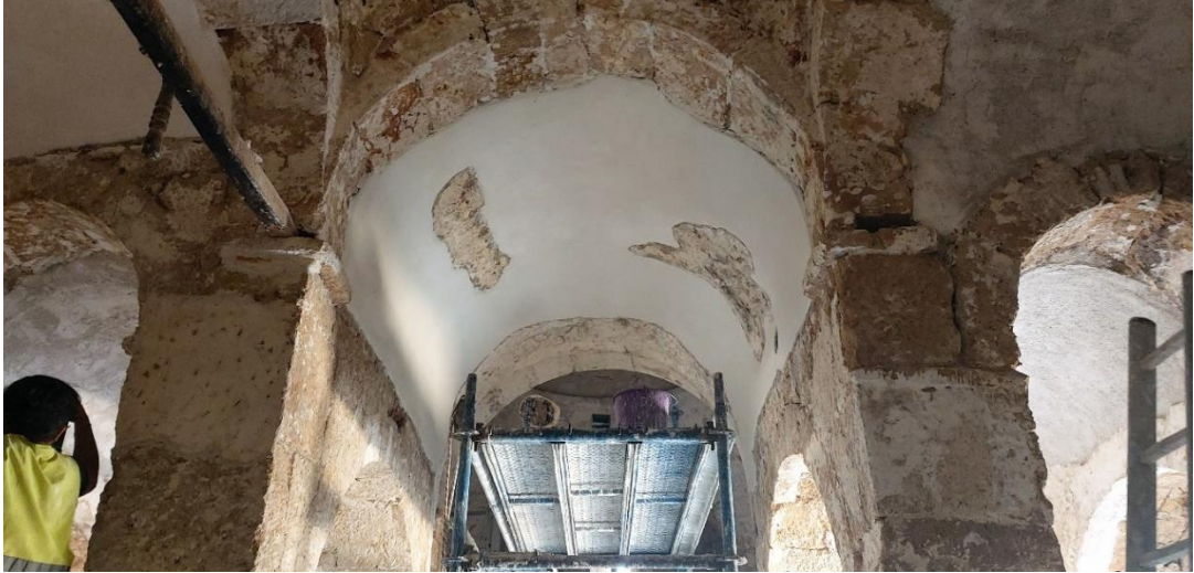
Figure 2.27: Final stage of plastering at ceiling
