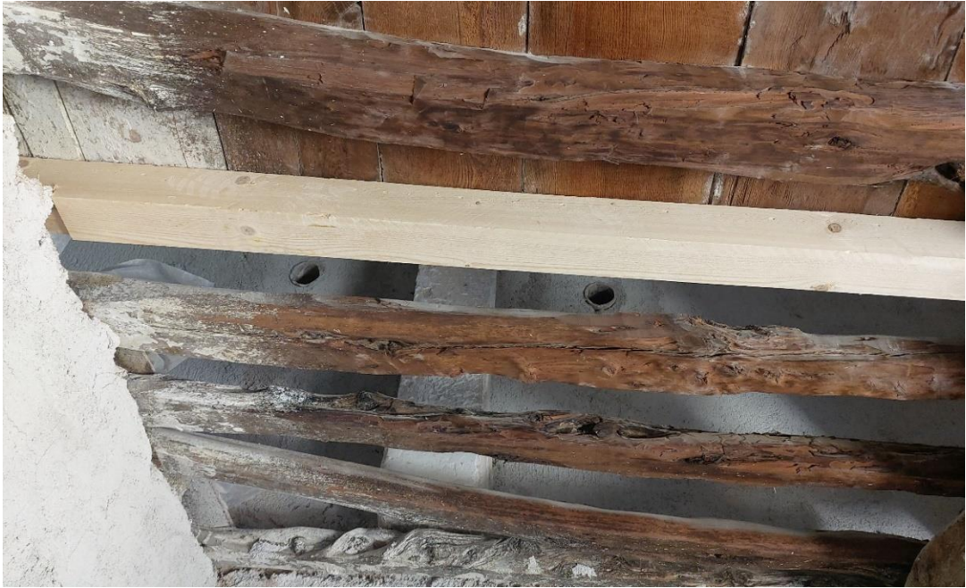
Figure 2.48: New wooden beam
