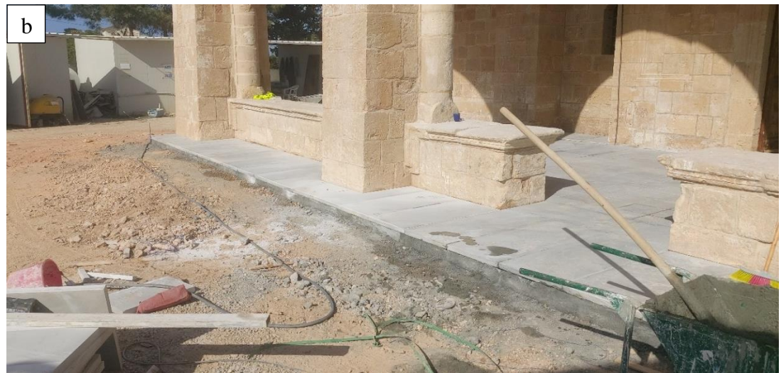
Figure 2.45: a) Construction of new floor with Local stone stage 1 b) Stage 2
