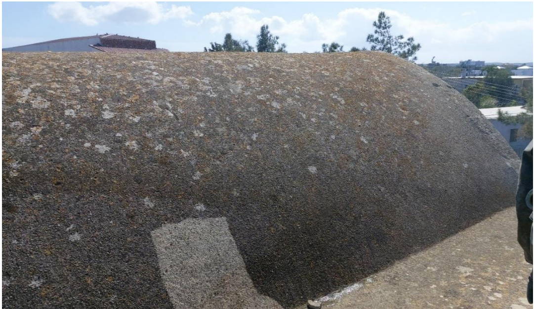
Figure 2.28: Cleaning of loose deposits stage 1
