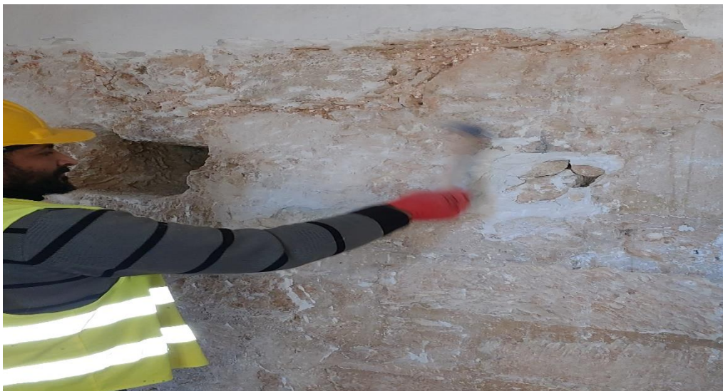
Figure 2.13: Cleaning of stone surfaces with brushes
