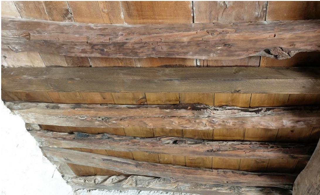
Figure 2.49: New wooden beam
