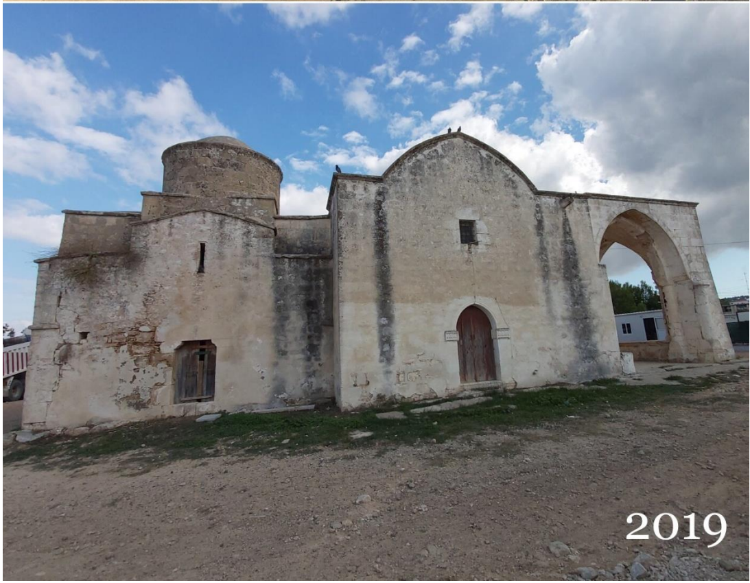
Figure 2.61: View of the west facade
