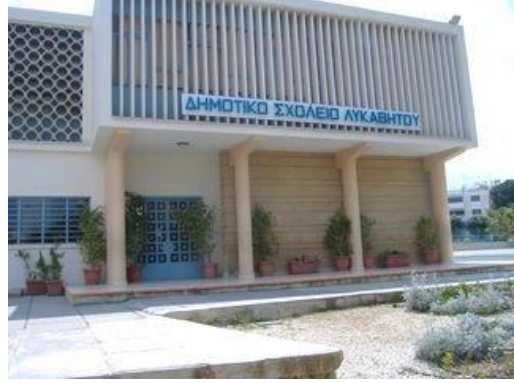
Figure 40: Vertically Arranged Brise-Soleil from Main Entrance View in Lykavitos Elementary School
