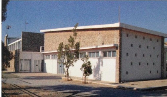
Figure 37: Single-pitch Roof in Lefkosa Technical School
