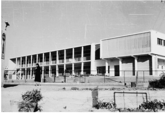
Figure 40: Vertically Arranged Brise-Soleil from Main Entrance View in Lykavitos Elementary School
