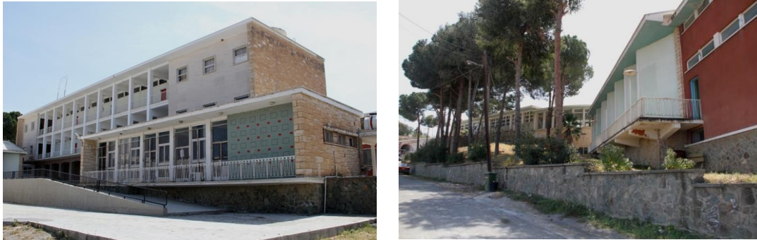
Figure 32: Cantilevered System in Lefke Technical School
