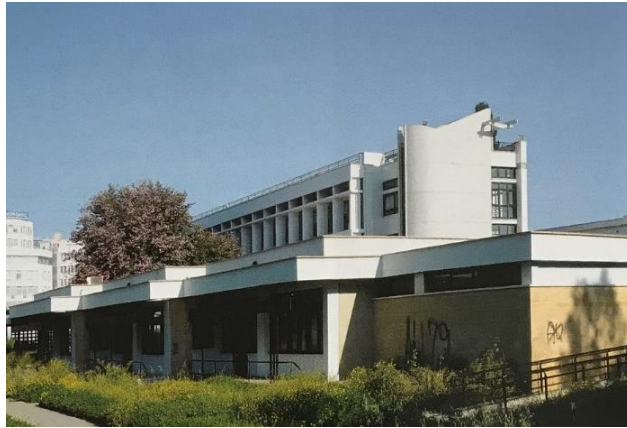
Figure 33: Vertical Shading Devices in Kykkos High School
