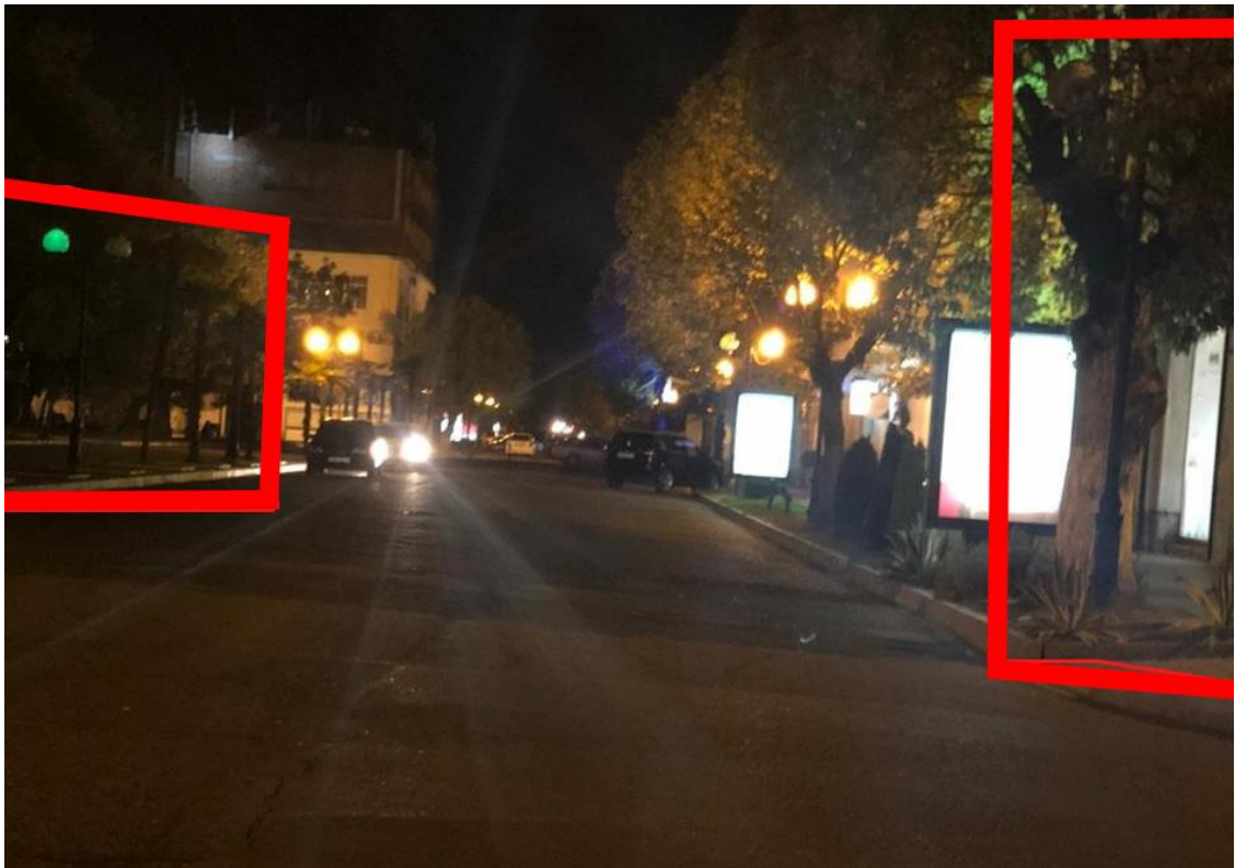
Figure 43: some lightings do not work and lighting close to the tree impedes proper illumination.
