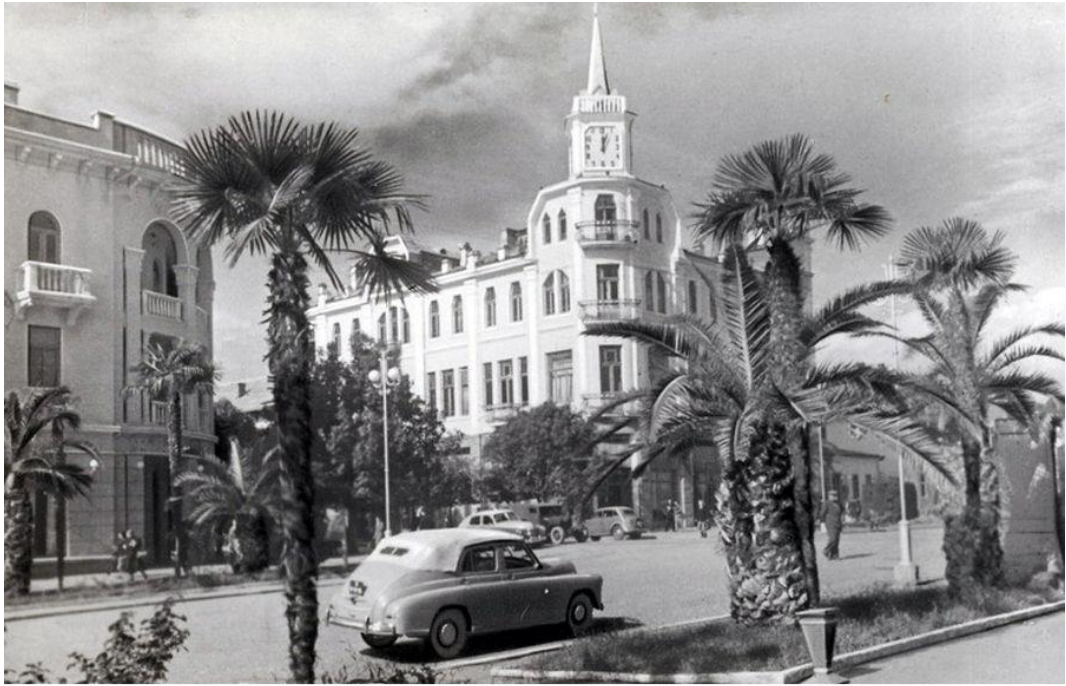
Figure 28: Administration building (retrieved from: Sputnik Abkhazia)
