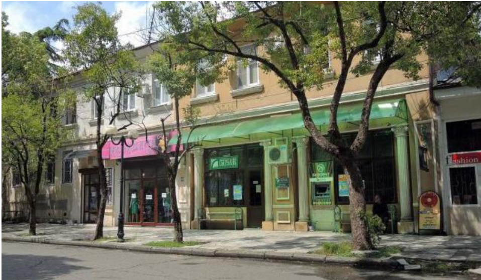
Figure 58: Violence of the appearance of the historic street.
