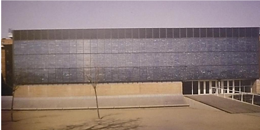
Figure 35: Pompeu Fabra Library, Spain, Mataro. View the south of the PV on double-skin façade (Robert and Guariento, 2009).
