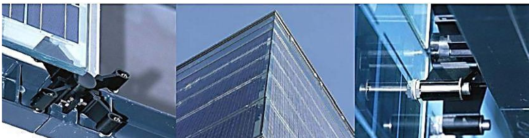
Figure 88: Detail of PV installation with point fixing and star-shaped as a support structure (Fischer Company, 2006)
