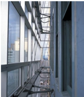
Figure 46: Air cavity of the structure of William Farrell Building, Canada, Vancouver http://www.perkinswill.com/work/telus-william-farrell-building.html
