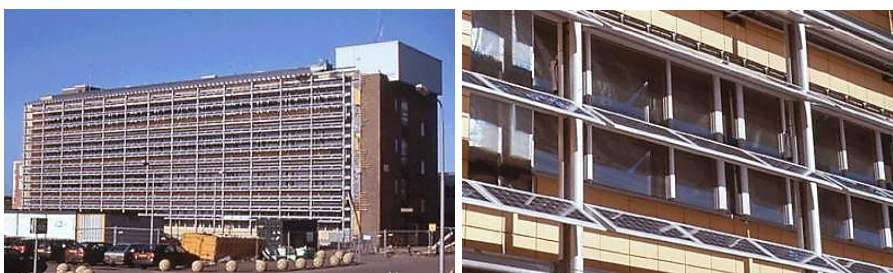
Figure 62: General view and detail of PV shading system of Energy Research Foundation (ECN) - Building 31 in Netherlands.
