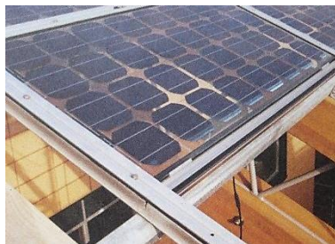
Figure 13: Monocrystalline PV in a semitransparent module (glass on the back) (Robert and Guariento, 2009)
