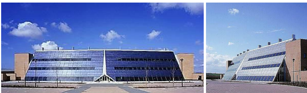
Figure 58: Solar Office, Doxford International Business Park, UK, Sunderland (Prasad D., Mark S, 2005).
