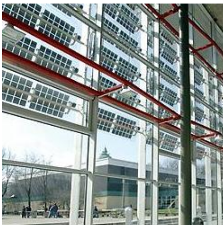
Figure 70: View from inside of extension of Goethe School http://www.ahnepohl-metallbau.de/
