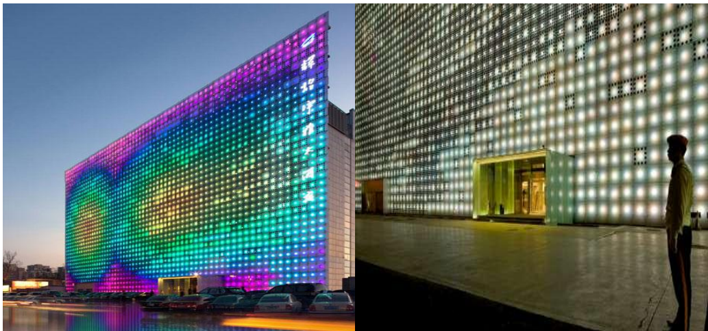
Figure 32: Xicui Entertainment Complex; an example lighting pattern at night of the LED array ( http://www.greenpix.org/download.php ).
