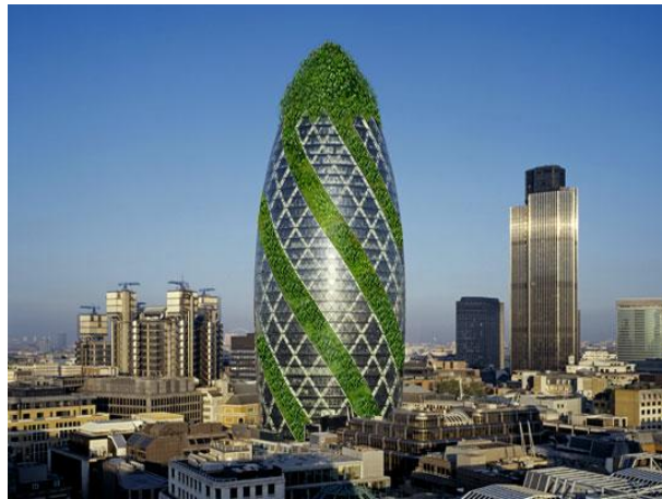
Figure 50: Sustainable iconic building (Gav)
