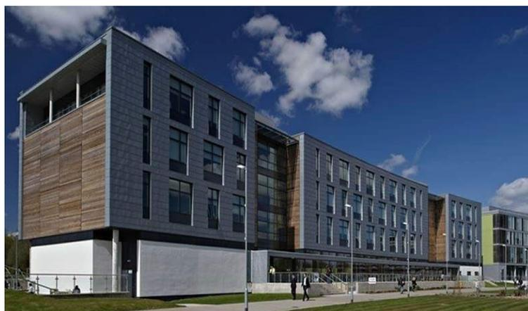
Figure 32: Building with Velfac composite window system.
