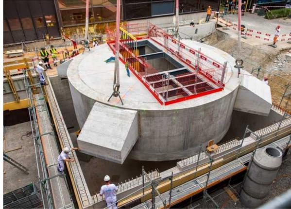
Figure 6: The concrete cylinder that encloses the centrifuge was already placed in August 2020.
