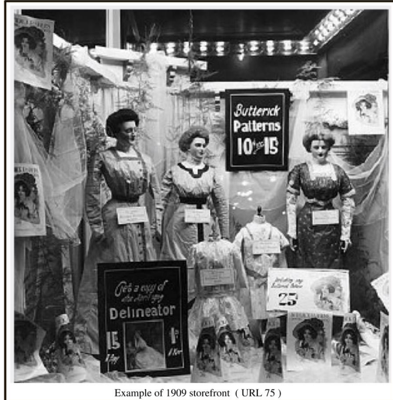
Figure 45: 1909 Storefront of Auerbach's Department Store in Salt Lake City, UT
