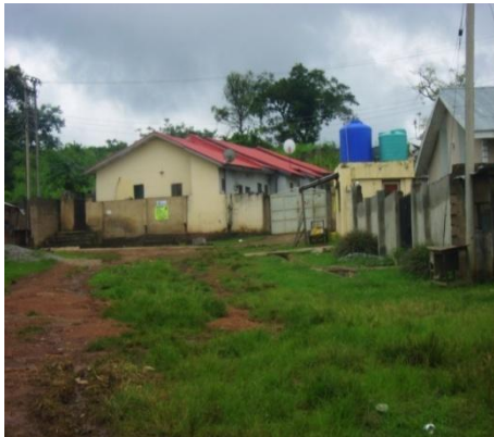
Figure 10: Quality of housing in one of the mass housing developments in Nigeria located at the outskirts of the city (Personal archive)
