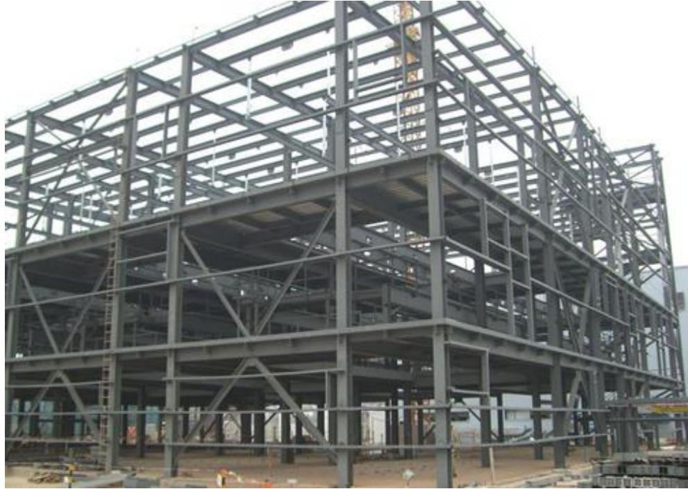
Figure 8: Steel building with columns, beams and bracing
