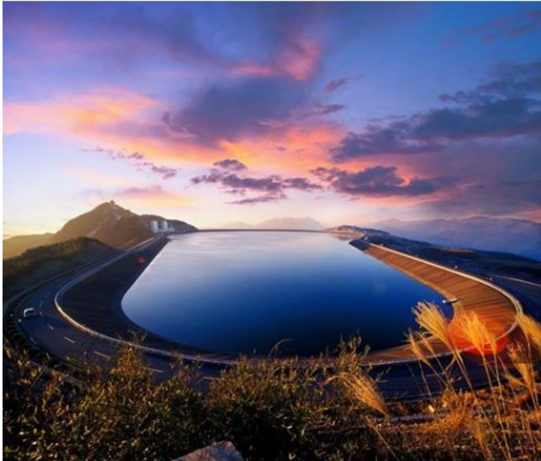
Figure 3. Tianhuangping pumped hydro storage reservoir (Zhejiang, China, 2016)
