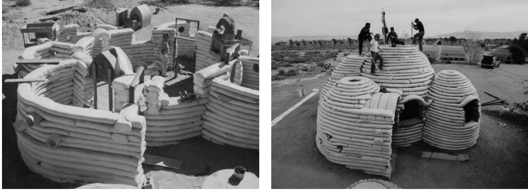
Figure 18: Earthbag unit structure. (Khalili, 2008)
