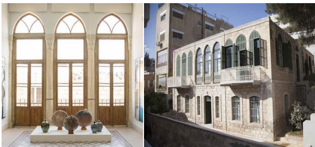
Figure 9: Using Arches in Doors and Windows in Old Traditional House & Covered the House by Stone (URL 4)
