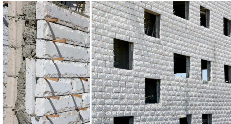
Figure 21: Fixing the Stone with Wooden Wedges (URL 16)
