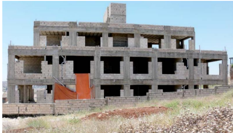
Figure 19: A structure House Built of Reinforced Concrete (URL 14)
