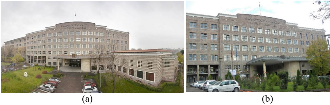
Figure 38: The Faculty of Languages, History and Geography (a) (Goethe-Institute Ankara. http://www.goethe.de/ins/tr/ank/pro/urbanspaces/web/philologie_2_gr.jpg ) and the Central Part of the Building (b) (Author, 2018).
