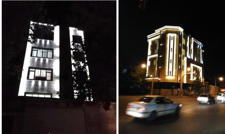
Figure 62: Exterior lighting of apartments in Mashhad. Source: author, 2017
