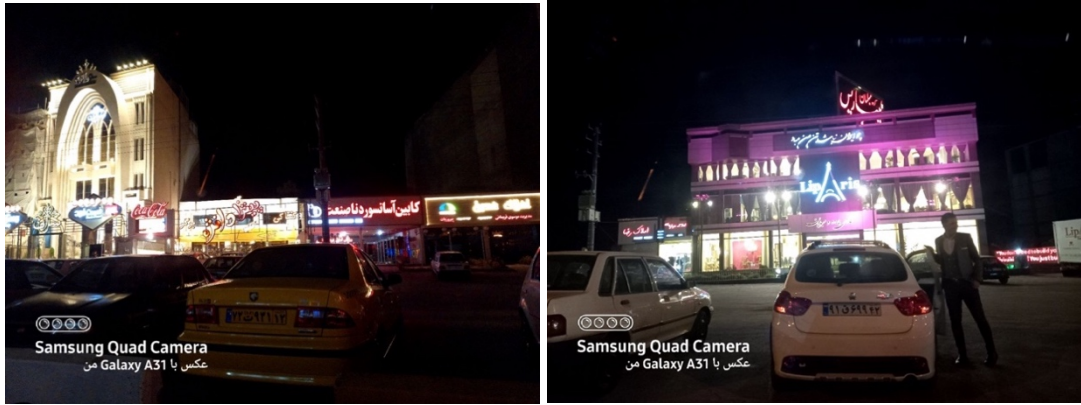
Figure 87: Facade lighting on buildings on the border of the city toward Torghabeh and Shandiz service cities
