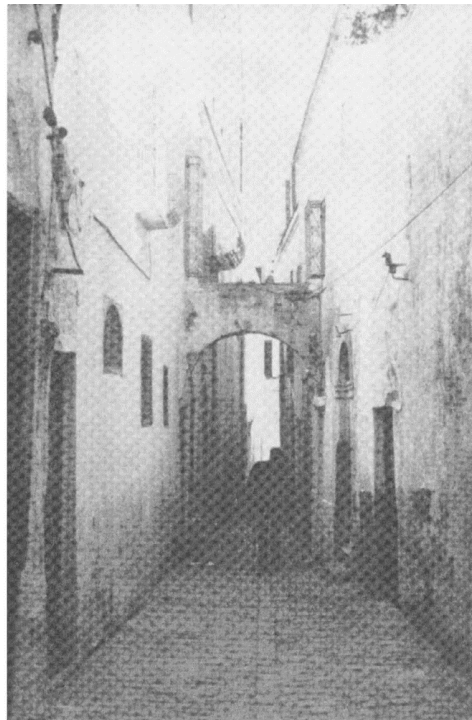
Figure 25: Windows are generally positioned above eye level on the street side, generally the threshold is nearly 1.75 m above street level (Hakim, 1986, p. 27)
