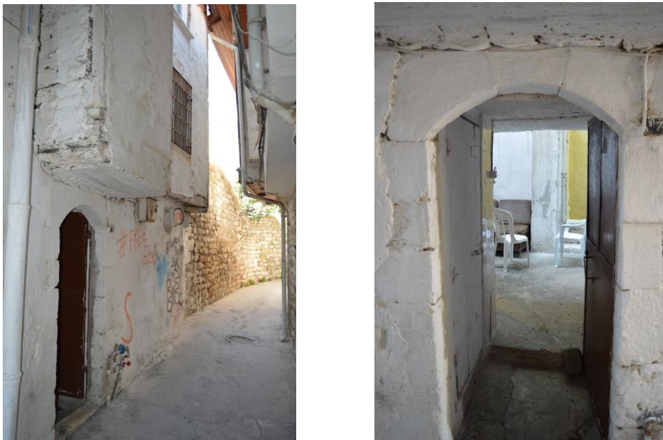
Figure 65: Entrance of House 75
