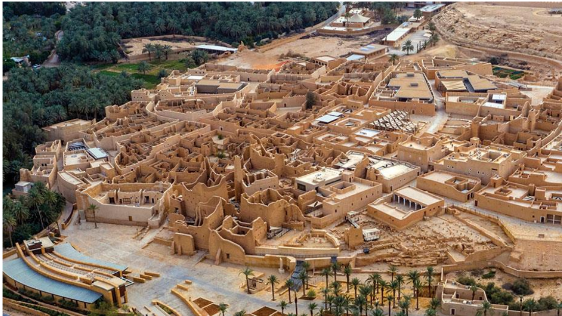
Figure 41: Bird's Eye View of the Historical At-Turaif District. Source - DDGA
