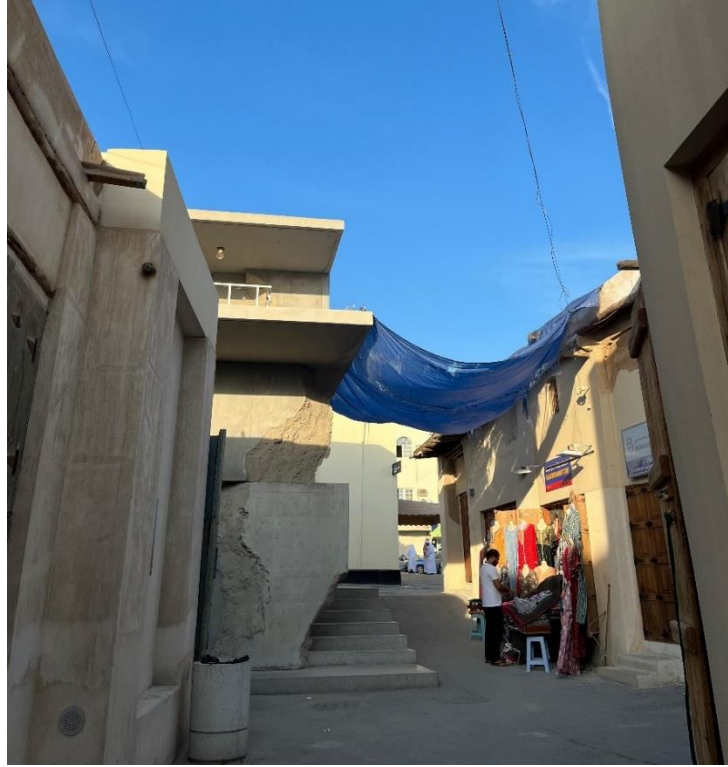
Figure 11: Muharraq's Regeneration Showing Replicating Authentic Facades. Source- Author
