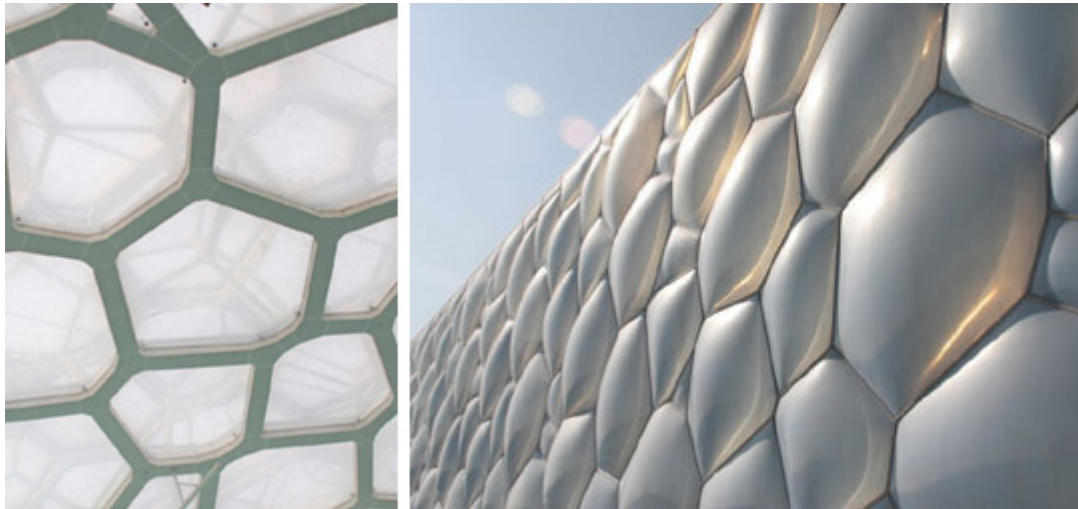
Figure 37: Usage of ETFE for Façade (Retrieved from: https://inhabitat.com/the-watercube-wins-australias-highest-architecture-award/ )
