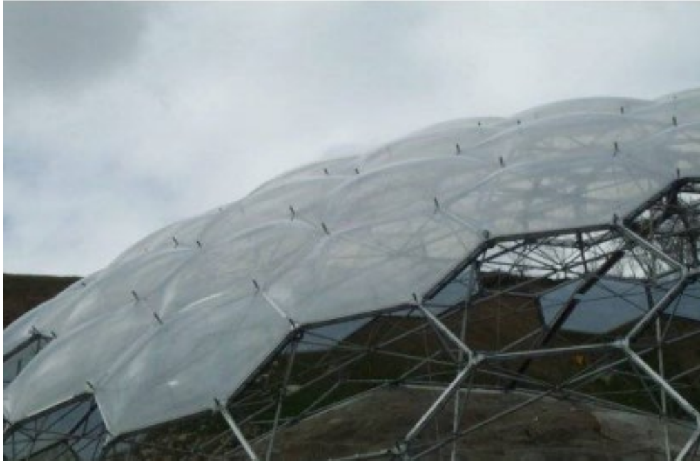
Figure 26: ETFE Pillows (retrieved from https://www.edenproject.com/eden-story/behind-the-scenes/architecture-at-eden )
