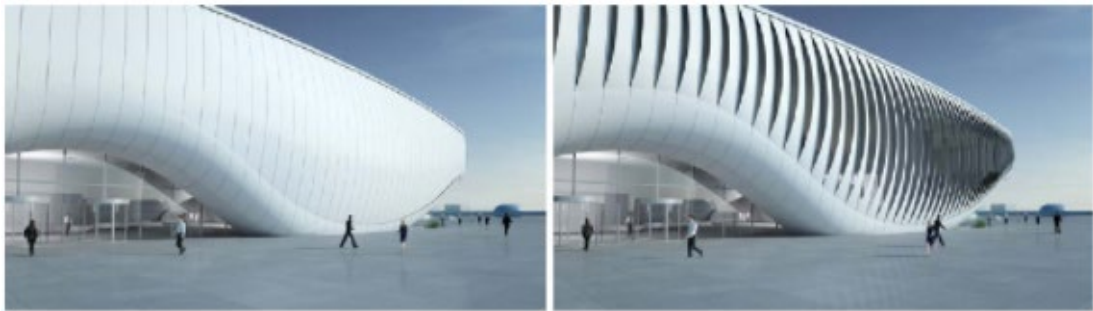
Figure 30: Movement of Louvers on Façade (Knippers et al.,2012)
