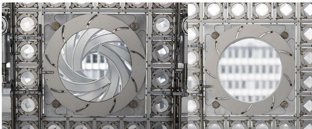
Figure 22: working mechanism of building envelope inspired from iris of the eye (Retrieved from https://www.imarabe.org/en/architecture )
