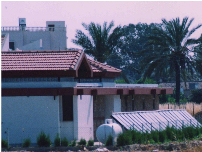
Figure.1 A house using solar collectors for underfloor heating, Nicosia, North Cyprus
